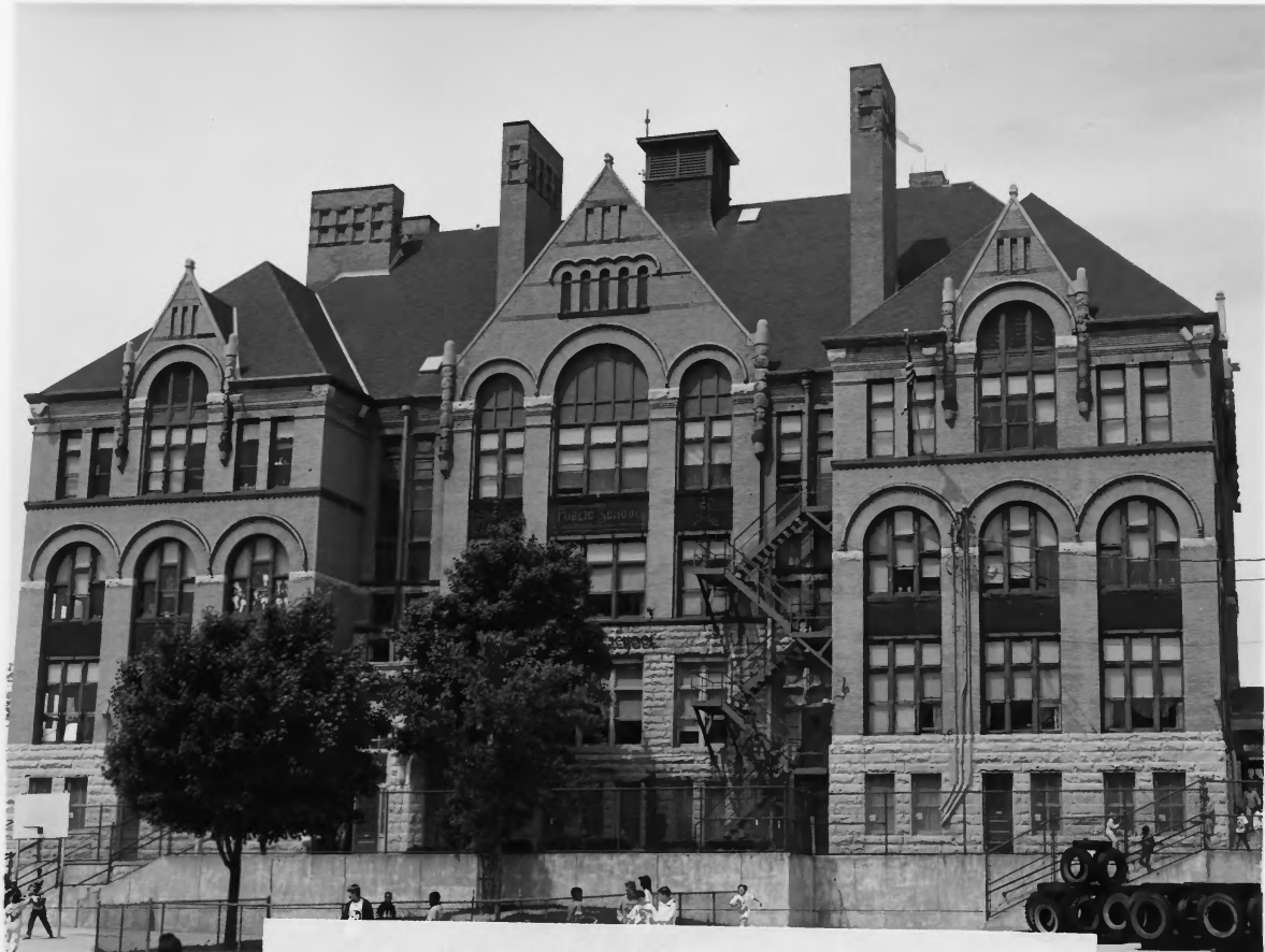
Fourth Street (Meir) School, Milwaukee, Wisconsin East facade Photo: Paul Jakubovich, 1990
