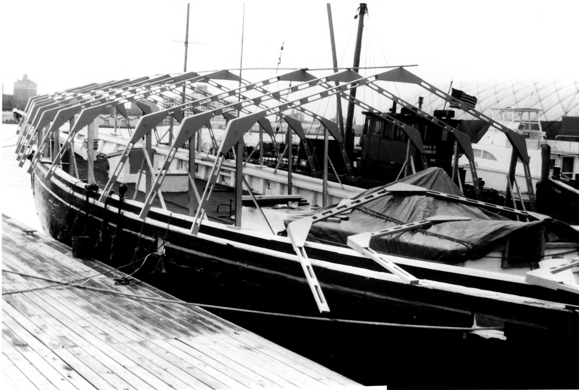
Lettie G. Howard , New York, New York. Photo provided by South Street Seaport Museum. South Street Seaport Museum, 1988. Lettie G. Howard Port stern Quarter at dock showing erection of protective "shiphouse". Photo # 4.
