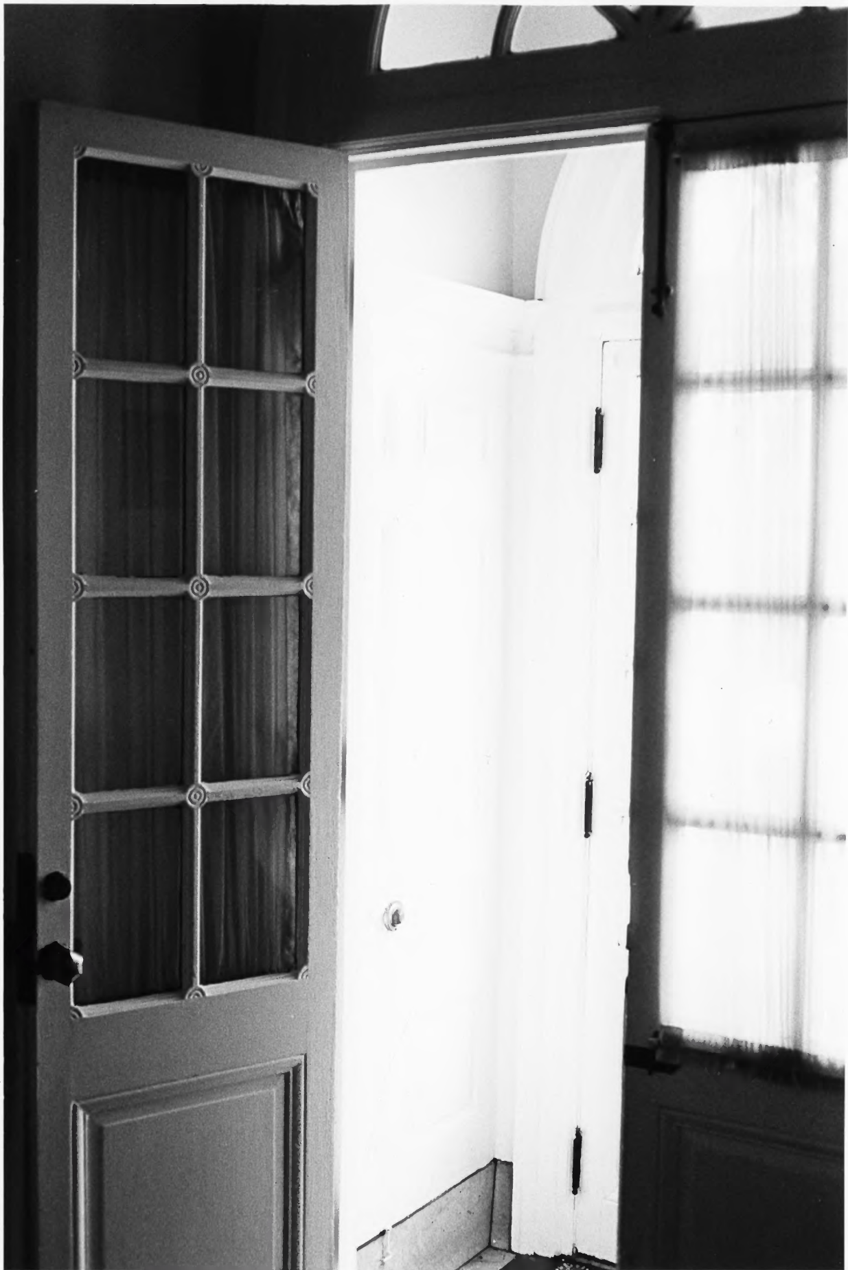
5/20 Interior, first floor, view of vestibule paneling and entrance doors
