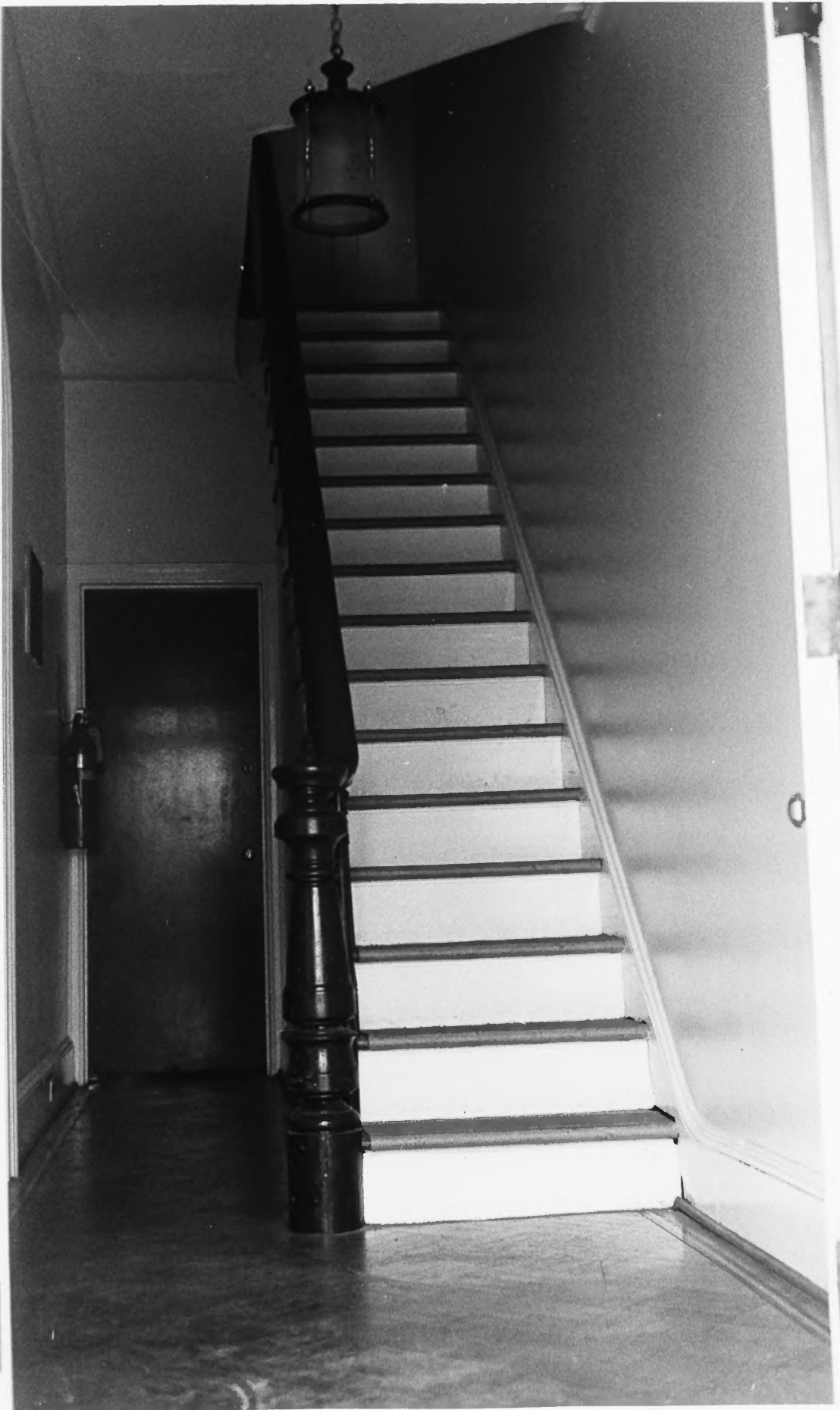
6/20 Interior, first floor, view of stairhall from vestibule, door at end of hall leads into back parlor
