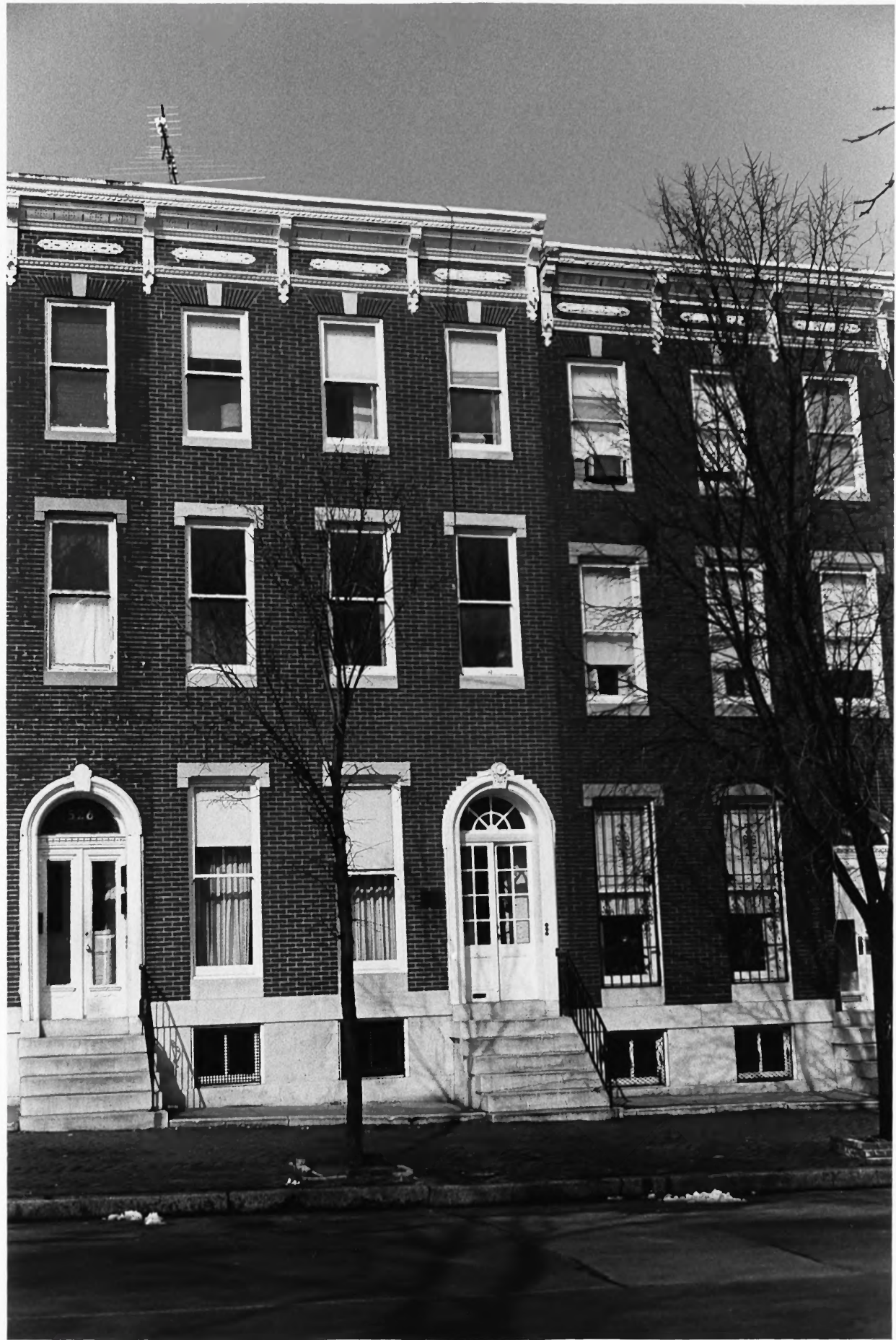
1/20 Facade or south elevation of house
