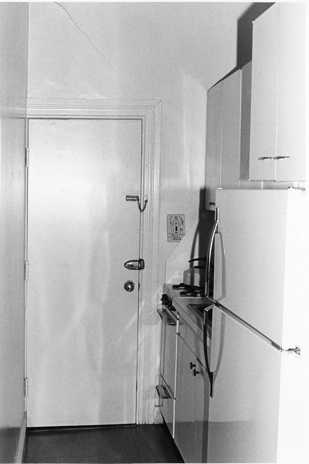
16/20 Interior, third floor, view of kitchen installed in el of front room, doorway leads into stair hall, partition on left was added when the kitchen was installed
