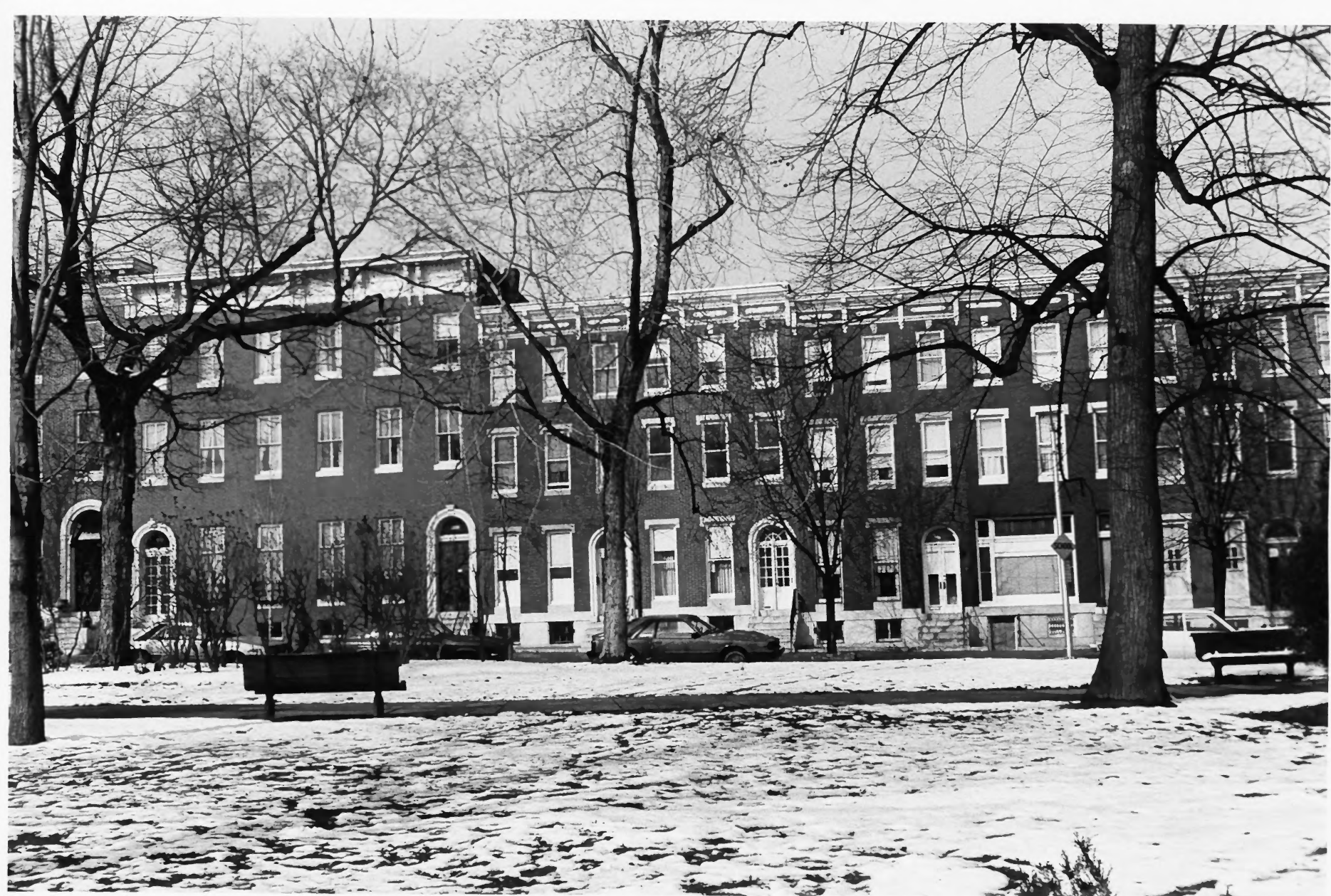
4/20 View of 1500 block of Hollins Street from Union Square with Mencken House in center of photograph
