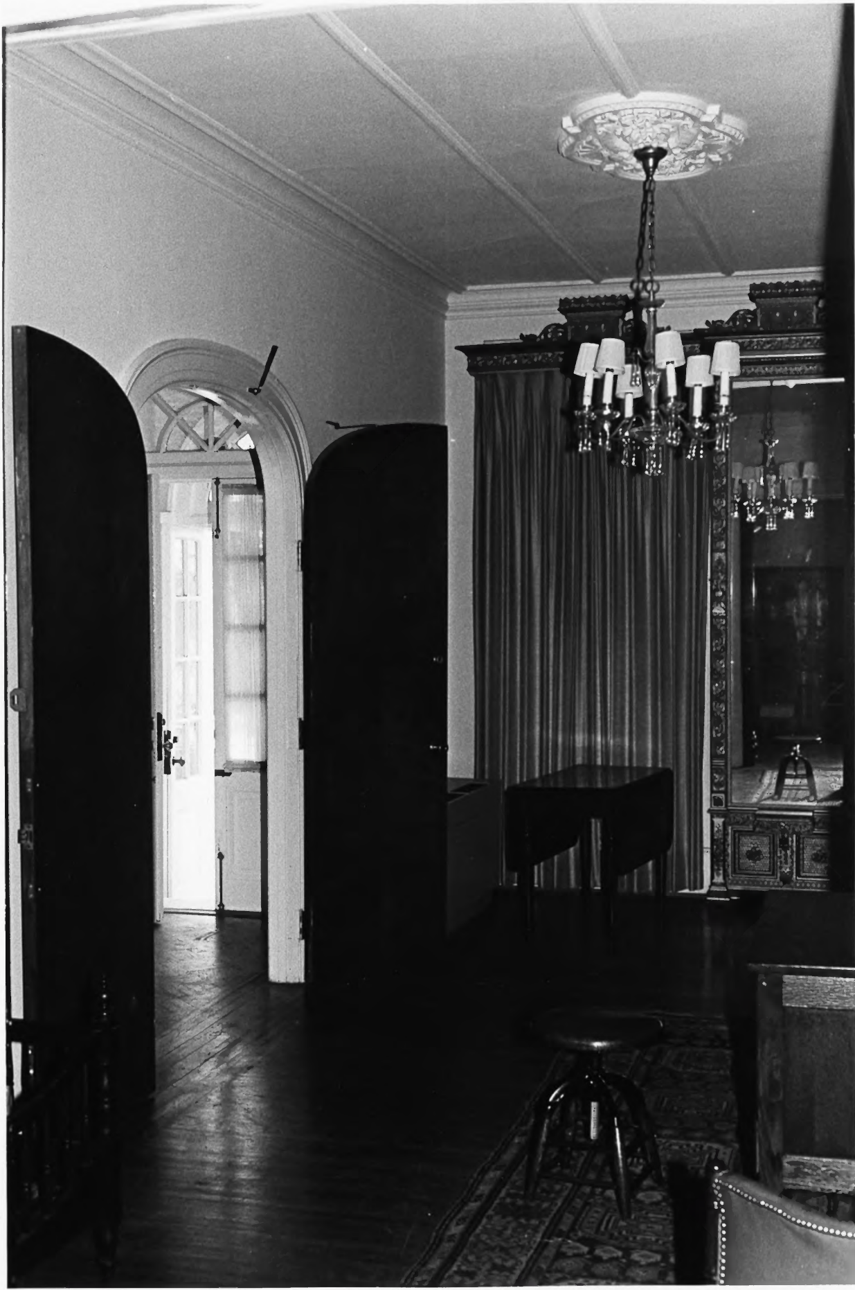
8/20 Interior, first floor, view of front parlor with hall and vestibule visible through arched doorway
