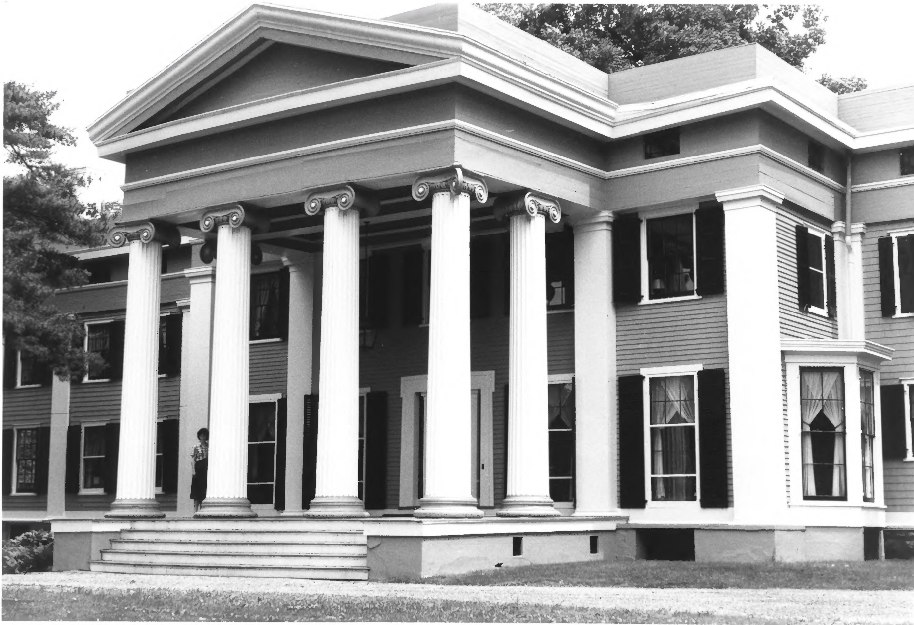
Boston Post Road Historic District, Rye, New York "Lounsberry" Facade
