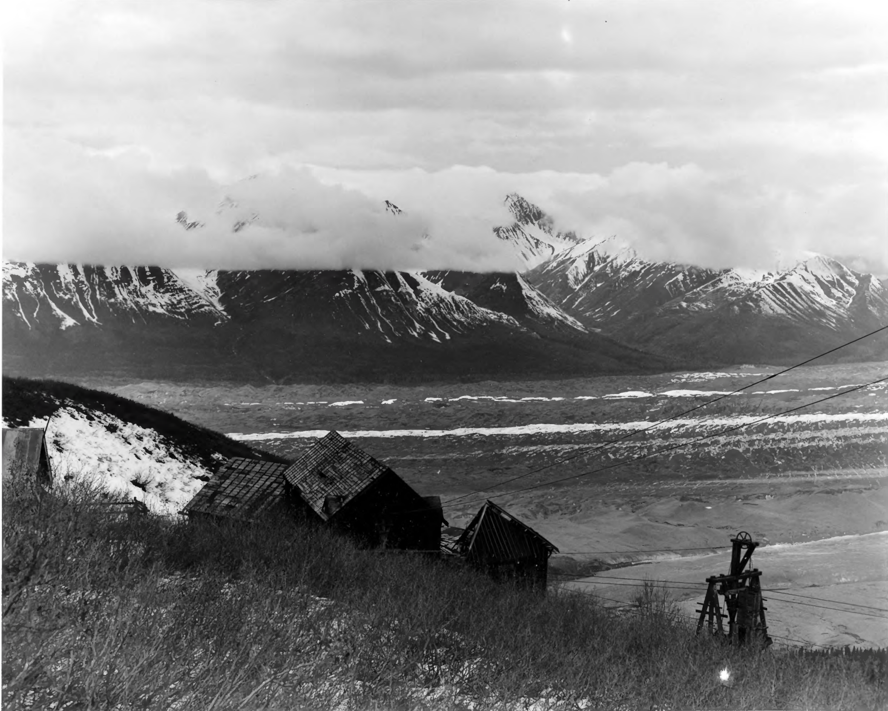
Kennecott Mines, mid-way tram buildings, Cordova-McCarthy Div., Alaska, U.S. Forest Service
