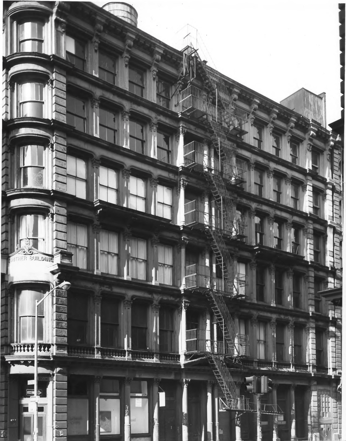
SoHo-Cast Iron Historic District, N.Y.
