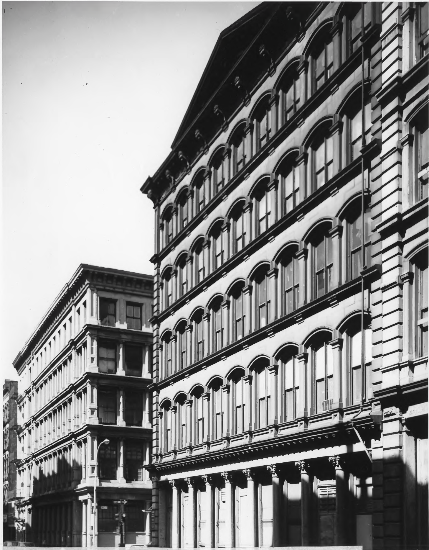
SoHo-Cast Iron Historic District, N.Y.
