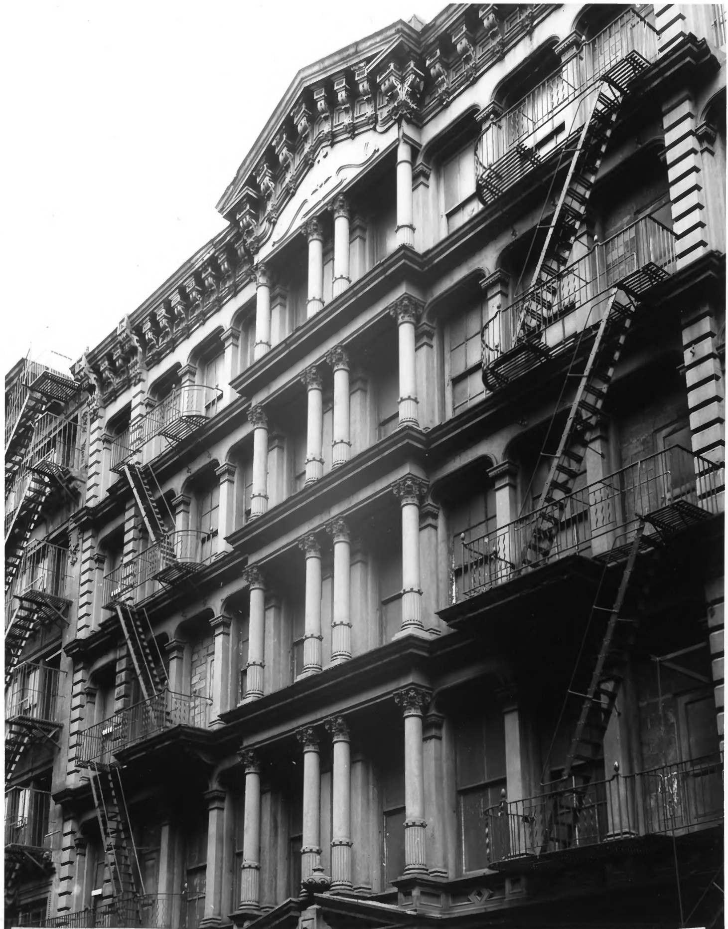
SoHo-Cast Iron Historic District, N.Y.
