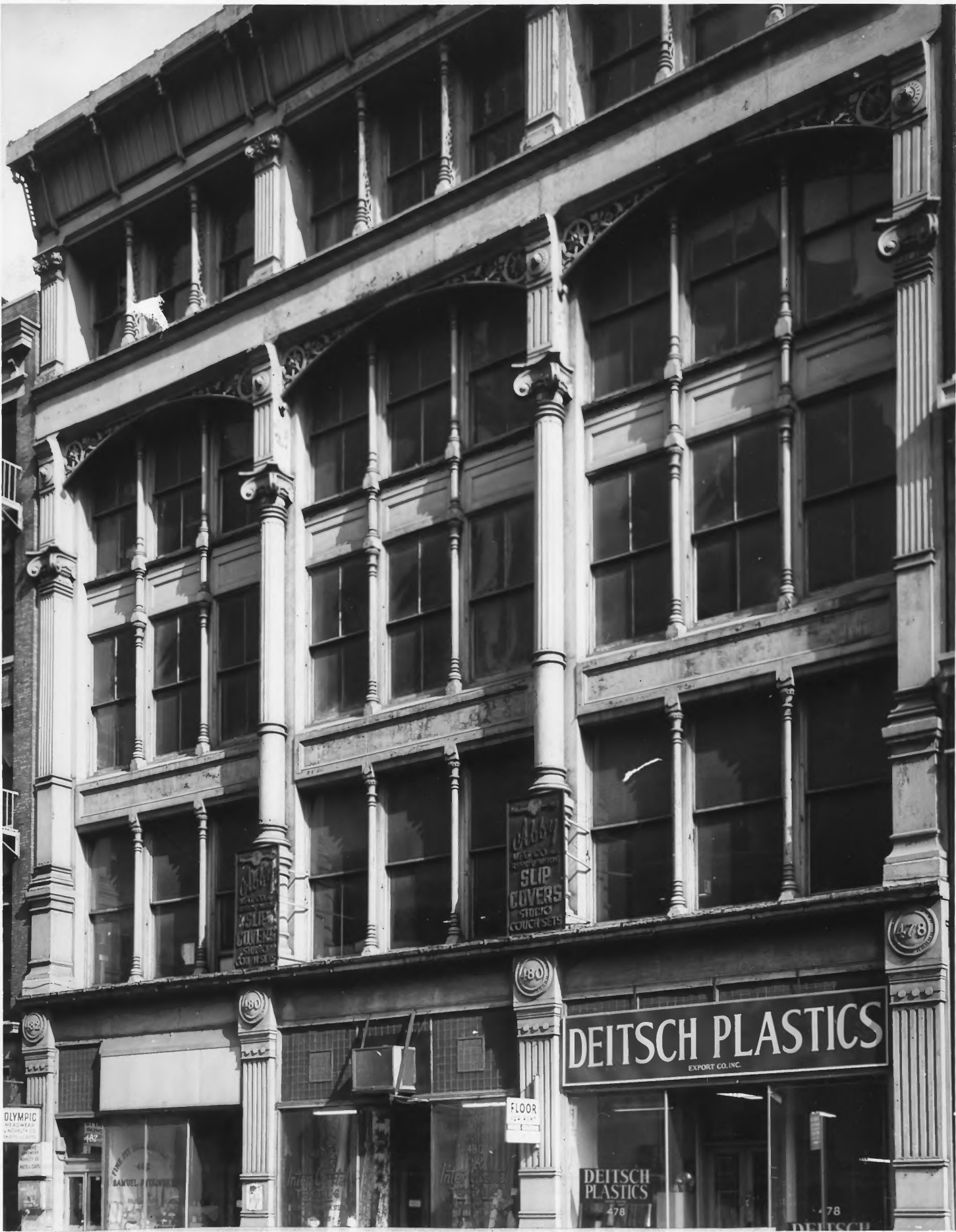
SoHo-Cast Iron Historic District, N.Y.
