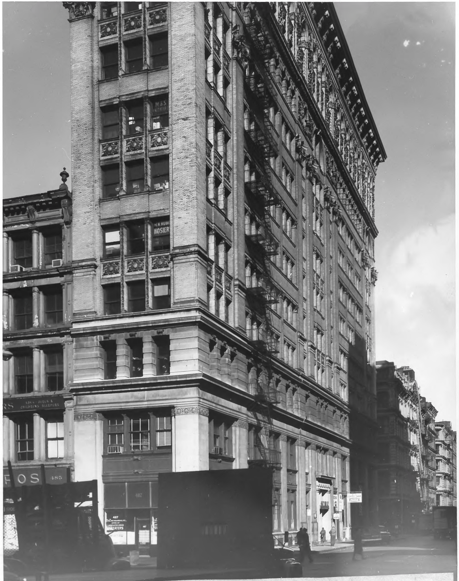
SoHo-Cast Iron Historic District, N.Y.
