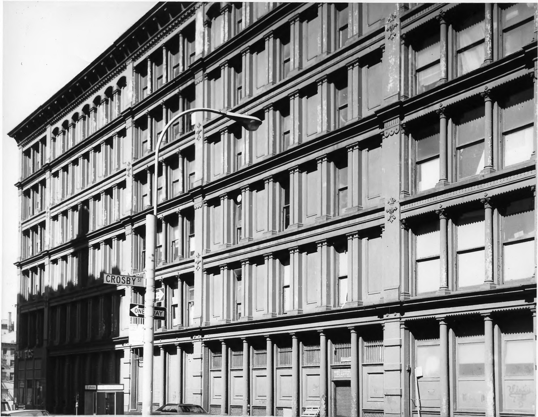
SoHo-Cast Iron Historic District, N.Y.
