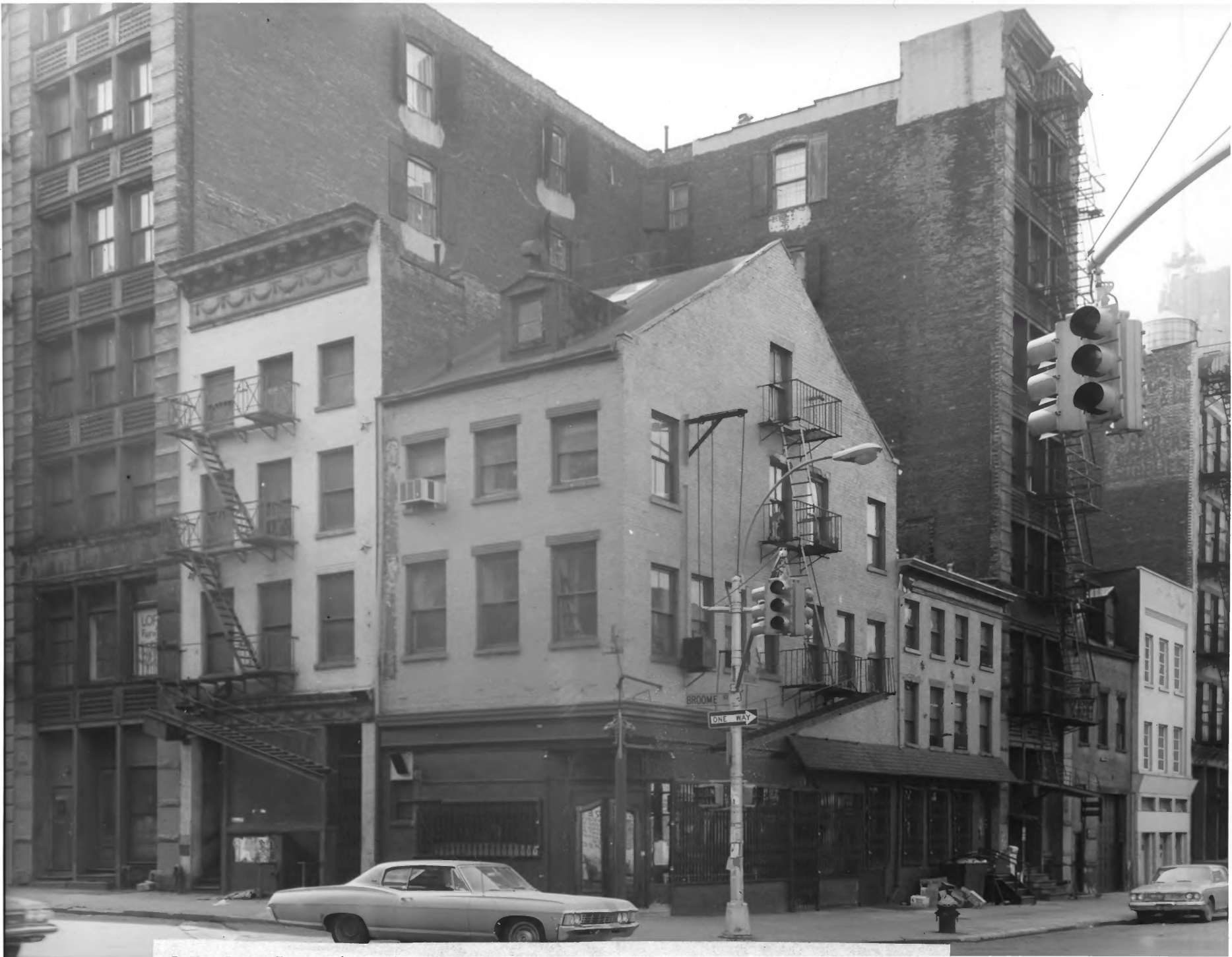
SoHo-Cast Iron Historic District, N.Y.
