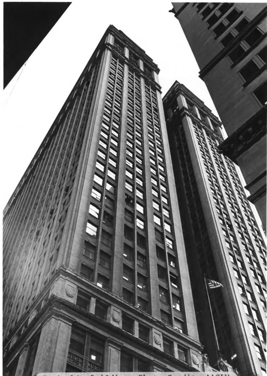
Equitable Building Photo Credit: AASLH
