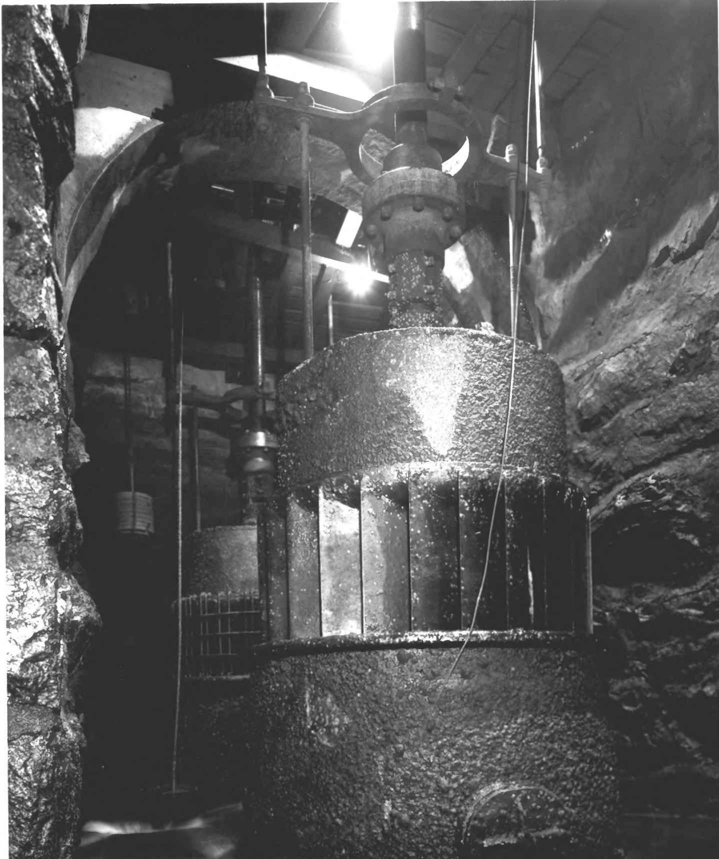
Eagle & Phenix Mills: Upper Power House Turbine #3.
