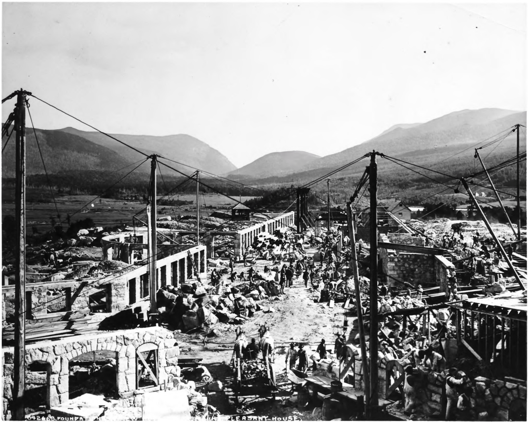
642468 FOUNDATION FOR THE BRIDGE AT PLEASANT-HOUSE.
