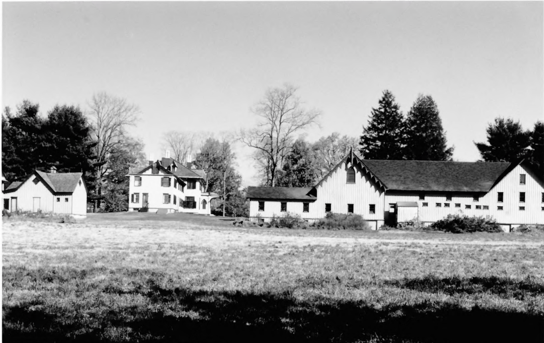
BOWEN, HENRY C., HOUSE (Roseland Cottage) Woodstock, Connecticut Ice house (left), west facade of house, barn & bowling alley (right) Photo by David Bohl, SPNEA, 1989
