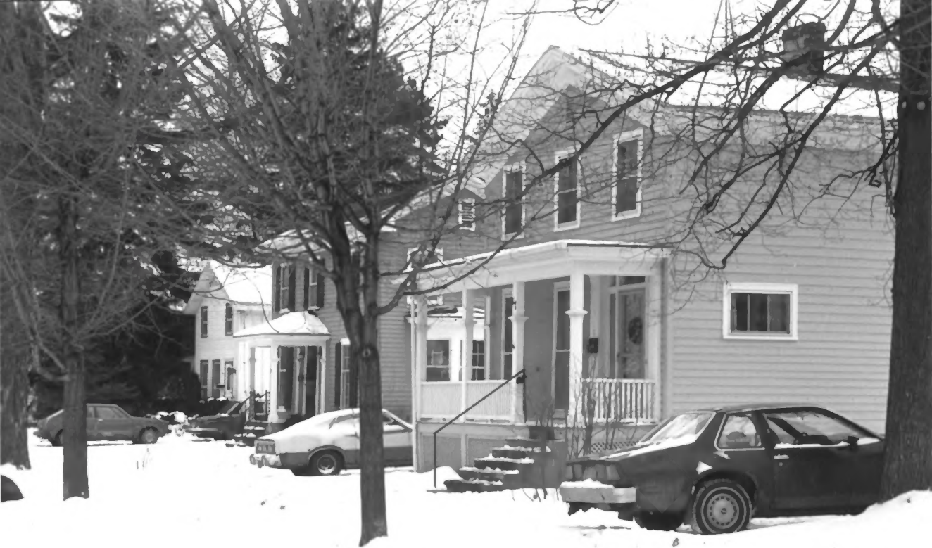
Geneseo Historic District Geneseo, New York 11-17 Elm St. Photo: APOG 1985 #43
