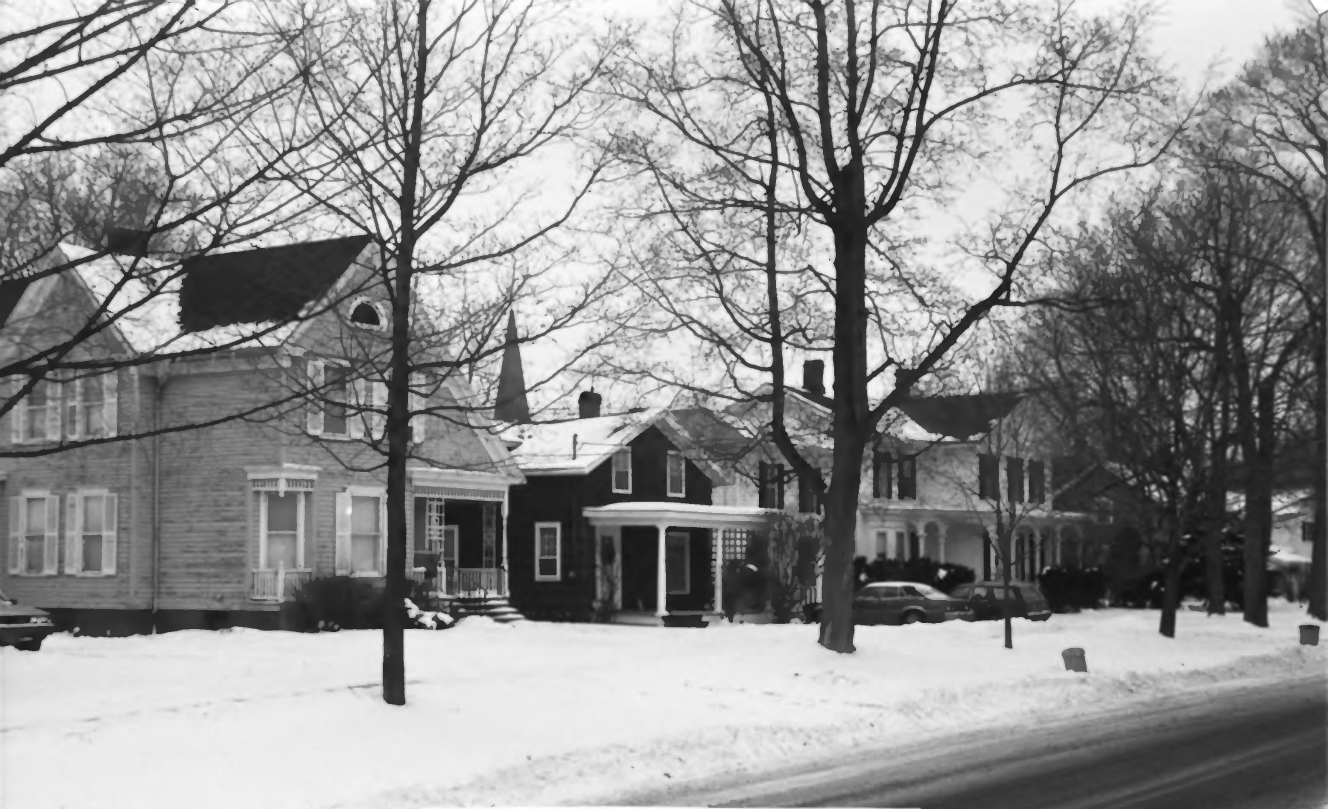
Geneseo Historic District Geneseo, New York 6-12 Second St. Photo: APOG 1985 #62
