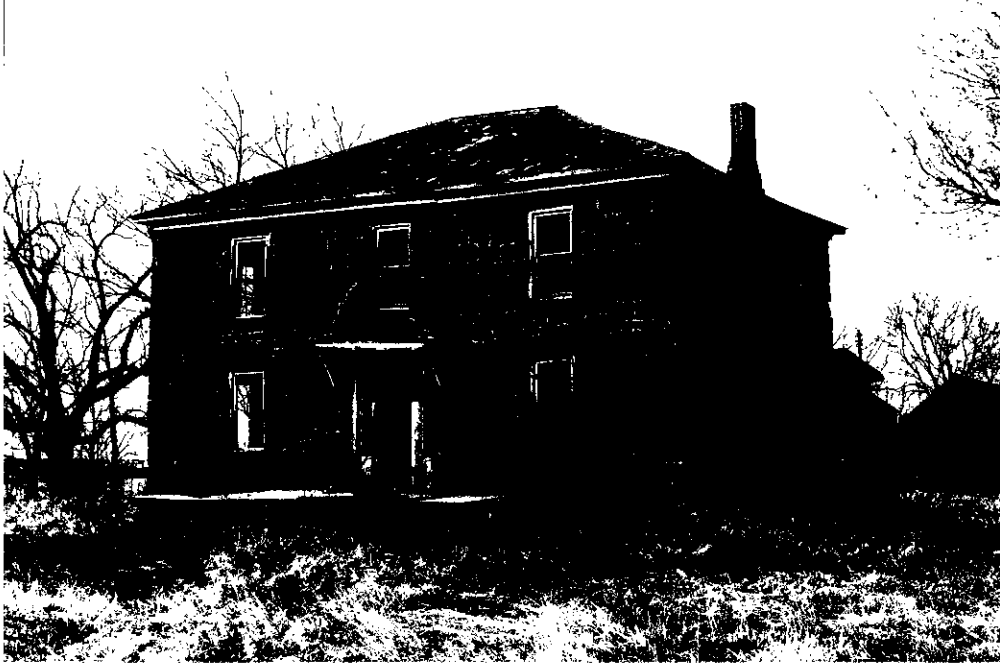
ca.1984 Photograph of Hitchcock House Prior to Restoration, View to the NNW
