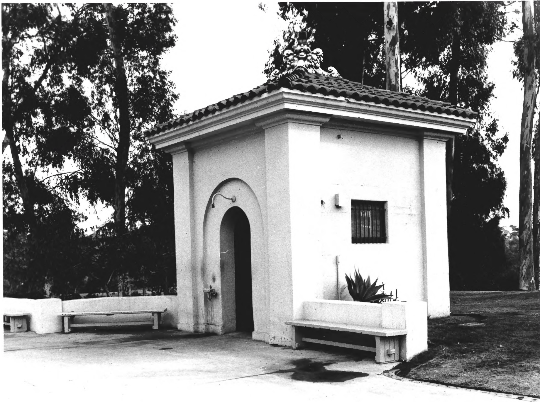
Cabrillo Bridge 1A. West Approach - Guardhouse on South Side of El Prado
