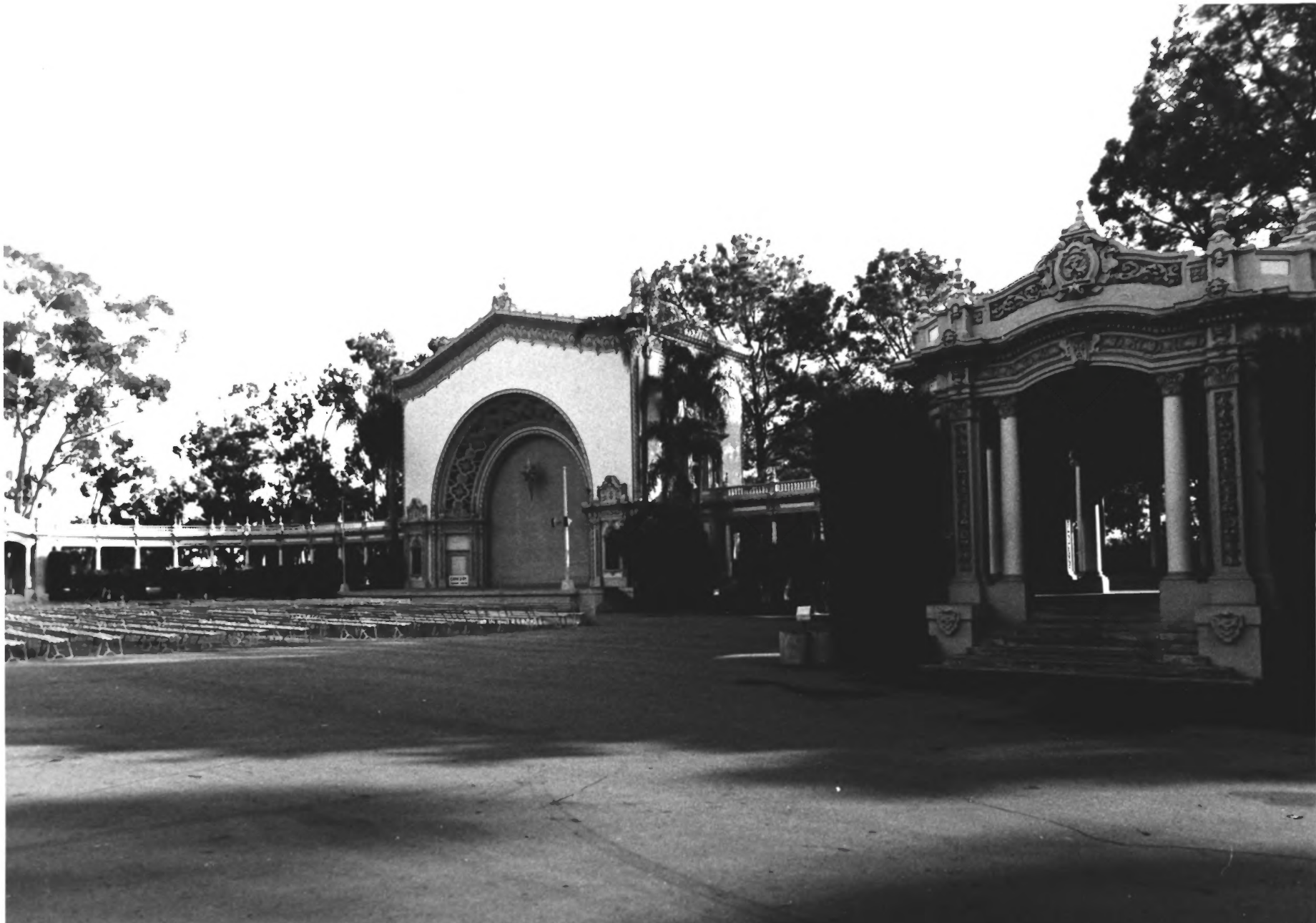
BALBOA PARK HISTORIC DISTRICT San Diego, California PHOTO CREDIT: City of San Diego DESCRIPTION: Organ Pavilion, View from Northwest
