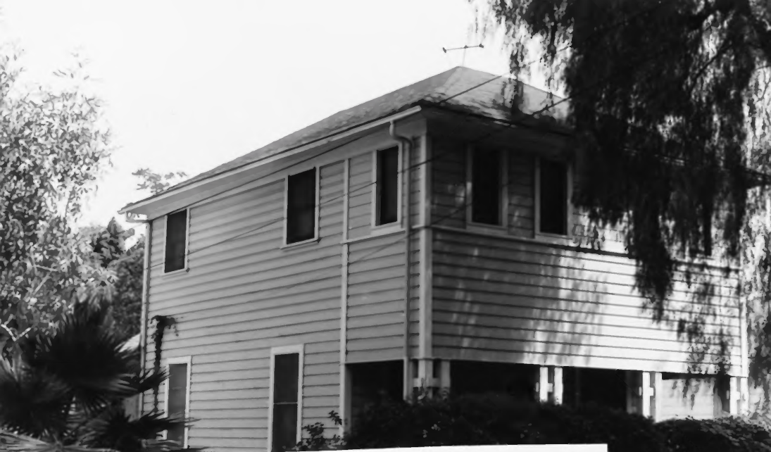
Harada House, Riverside, California Street facade Photo: Allan Curl, Riverside Museum, 1990
