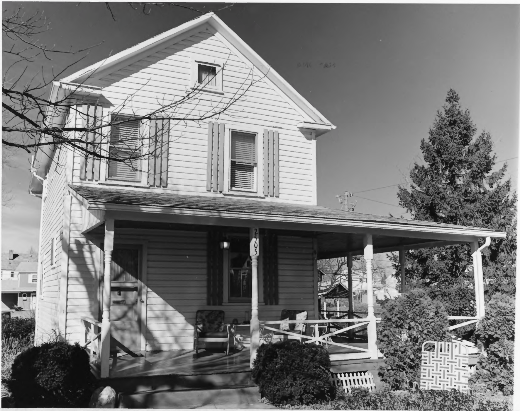
Charles Richard Drew House, Arlington, Virginia South elevation looking north
