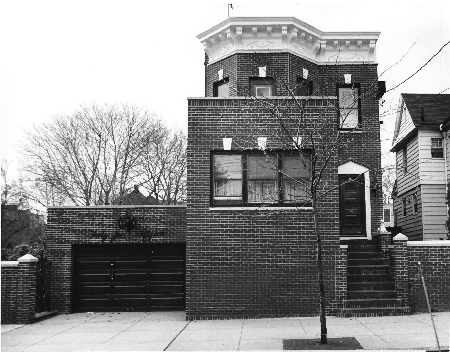
Louis Armstrong House, Corona District, Long Island, New York Photo by Richard K. Dozier for ABC 1975 Front elevation, looking east.
