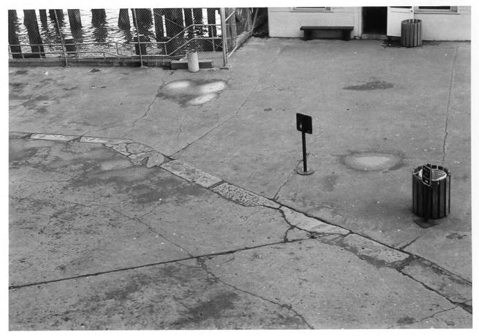
THE WHARF, SHOWING A STONE BULKHEAD BUILT 1874 OUT OF THE PLATFORM STONES OF AN 1850'S GUN BATTERY.
