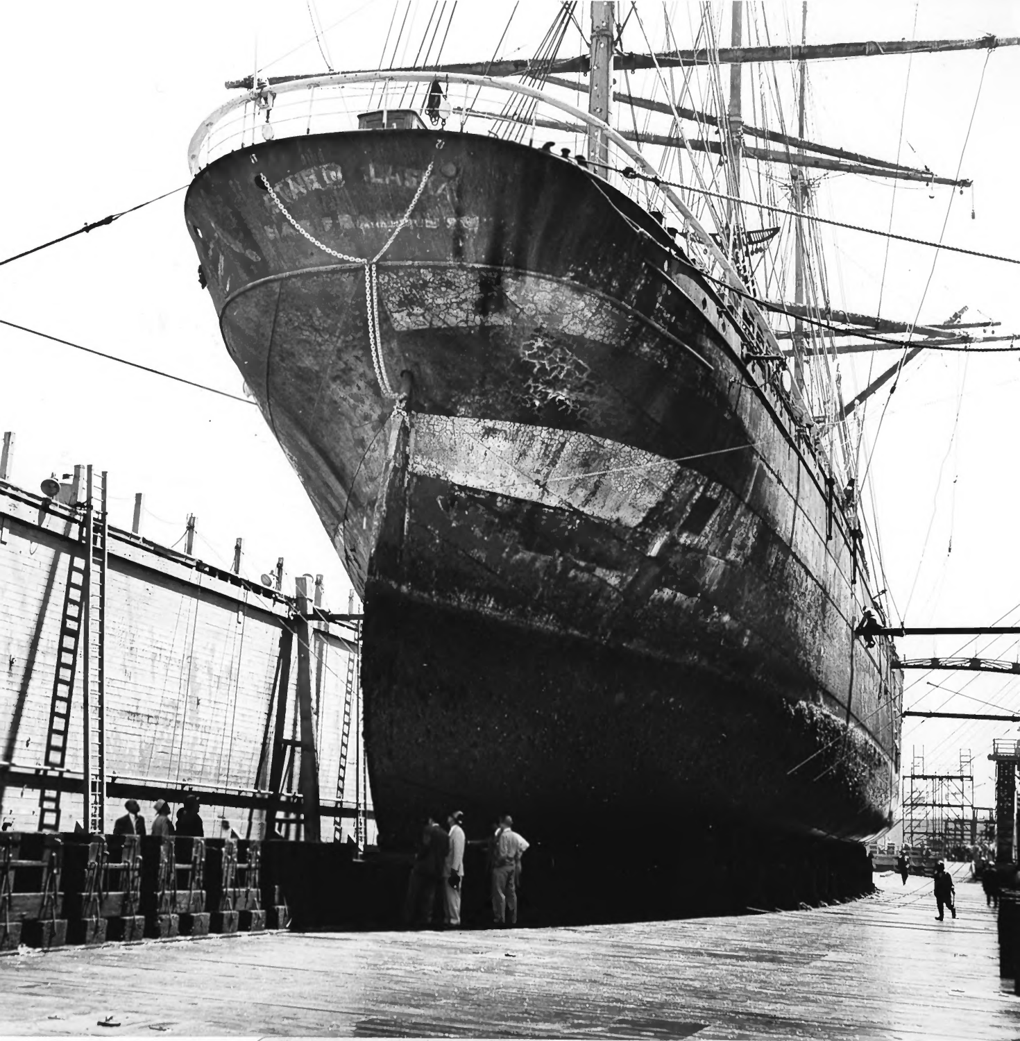
Balclutha as Pacific Queen , in drydock during restoration, 1954-55 San Francisco Bay area, California National Maritime Museum, San Francisco, photograph B4.35,640n
