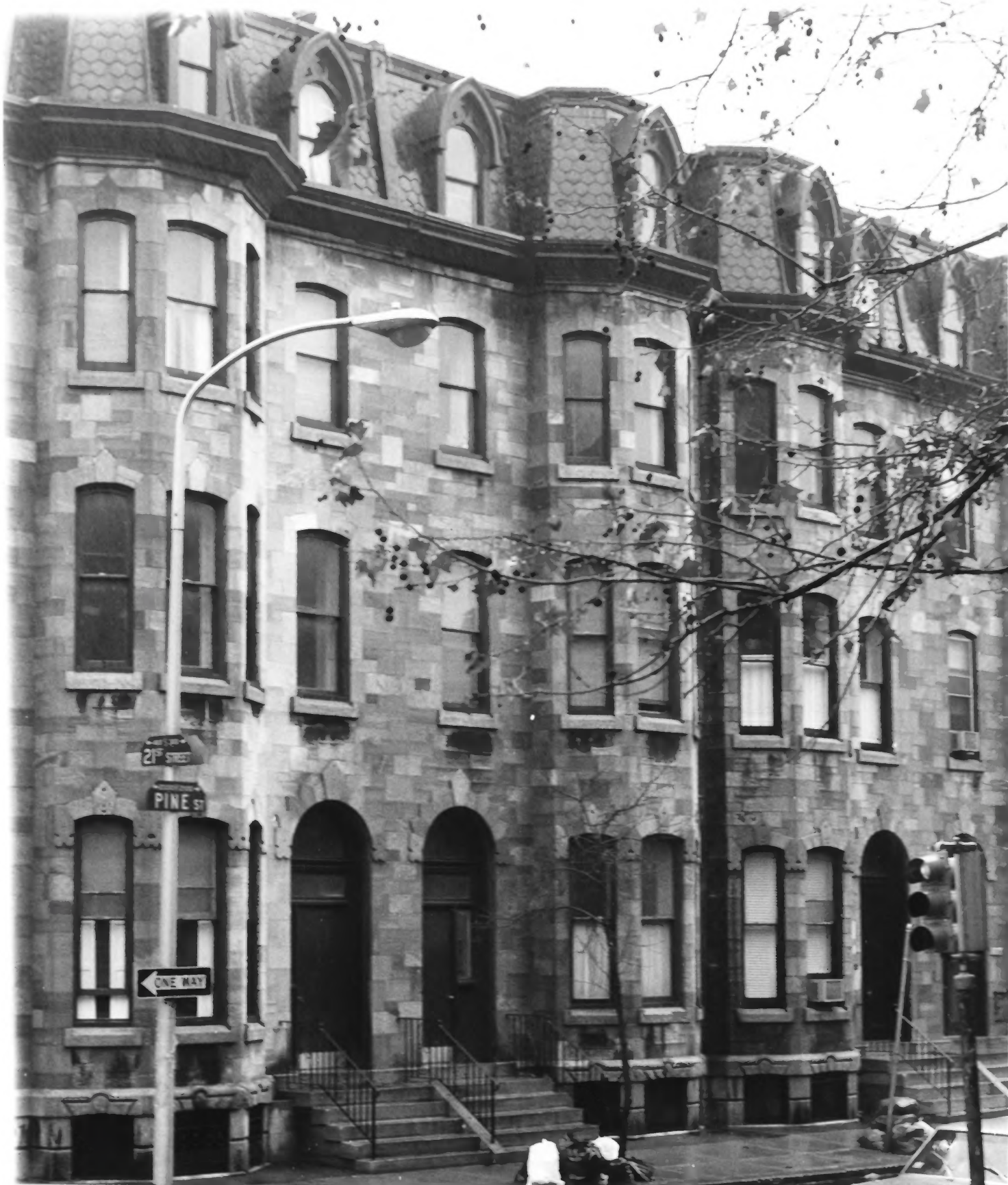
Edward D. Cope House, Philadelphia, Pennsylvania
