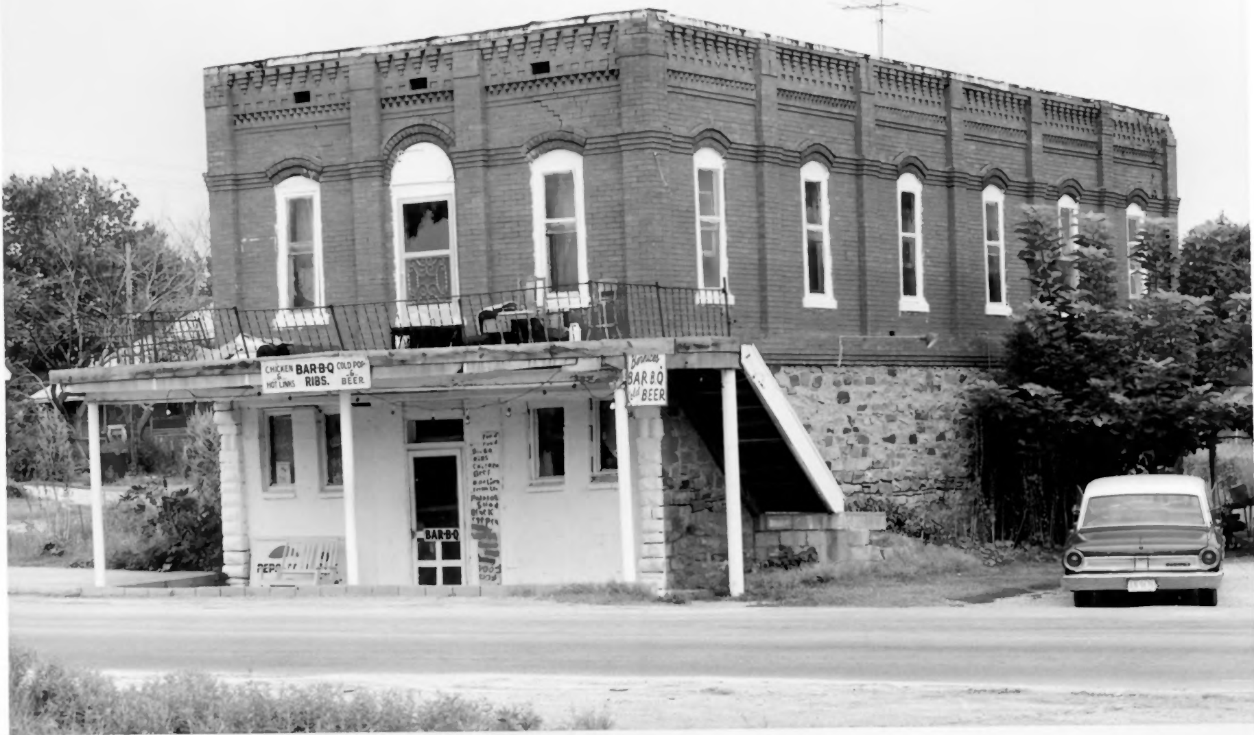
Boley Historic District (Boley Bank and Trust Company), Boley, Oklahoma Photo by Myers Commercial Photo for ABC and NPS, 1974
