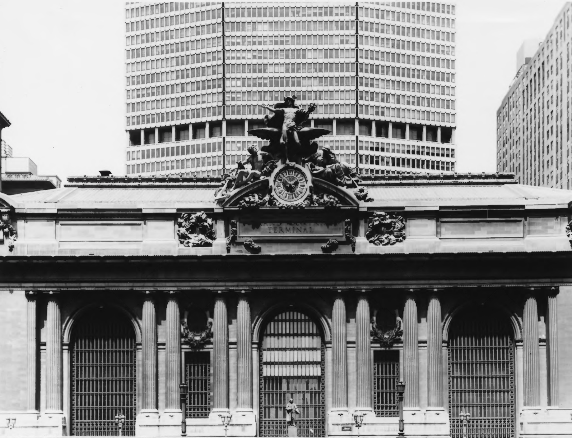
Grand Central Terminal
