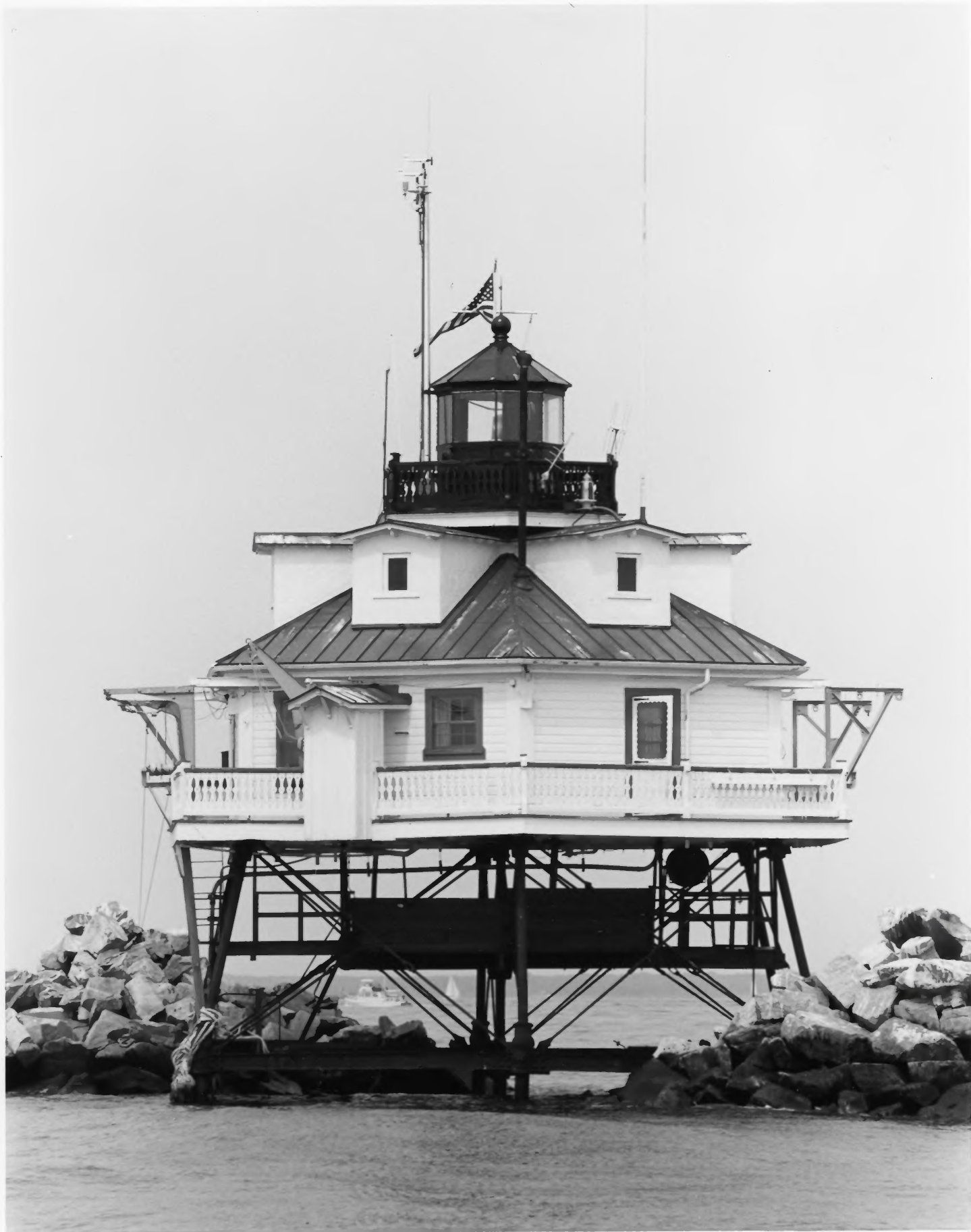
Thomas Point Shoal Light Station Near Annapolis, MD Tower in 1990 U.S. Coast Guard Photo by R.B. Ressler
