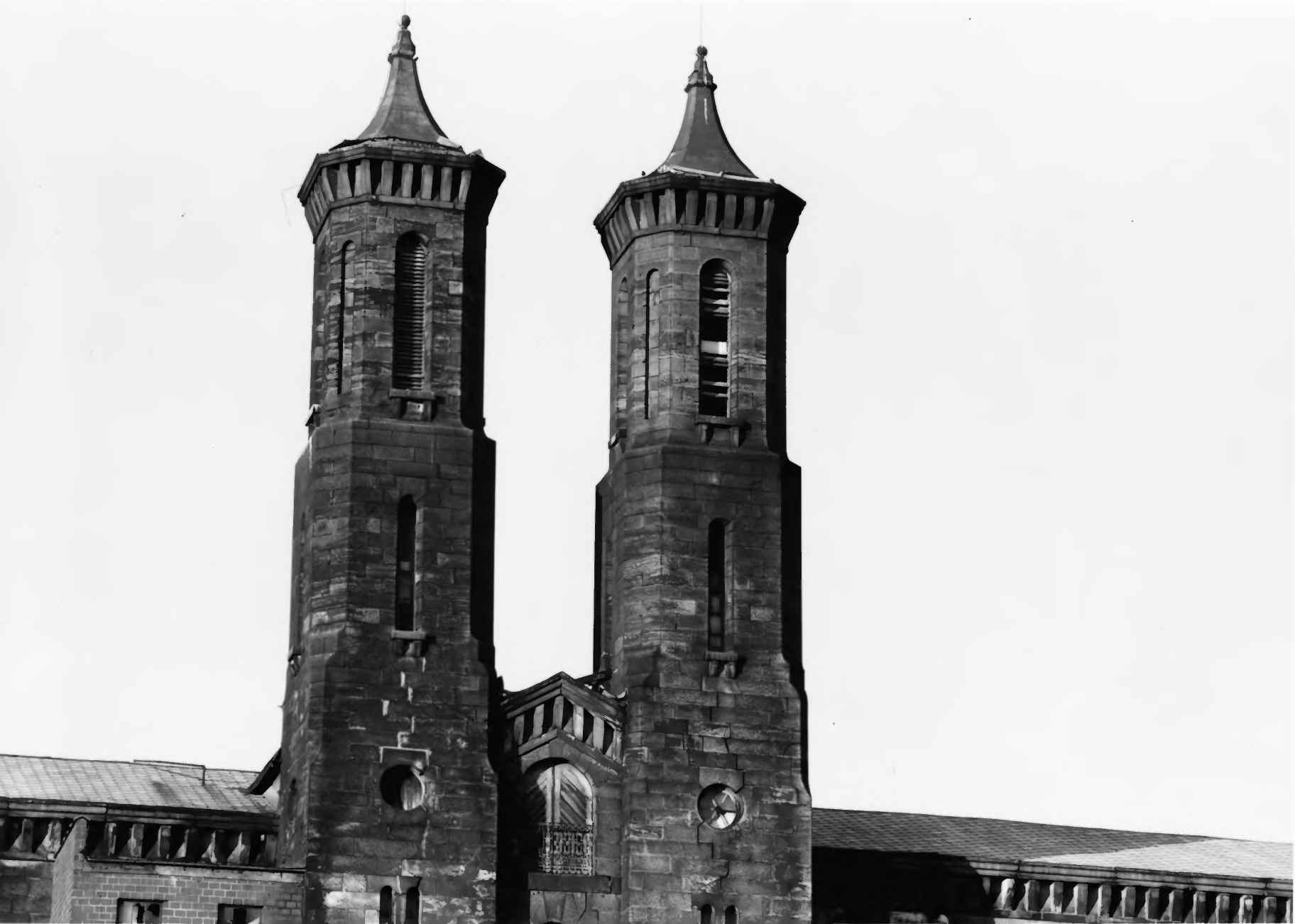
7. CANNELTON MILLS, INDIANA Detail, Telephoto of Twin Towers Photo: Boucher, HAER, 1974
