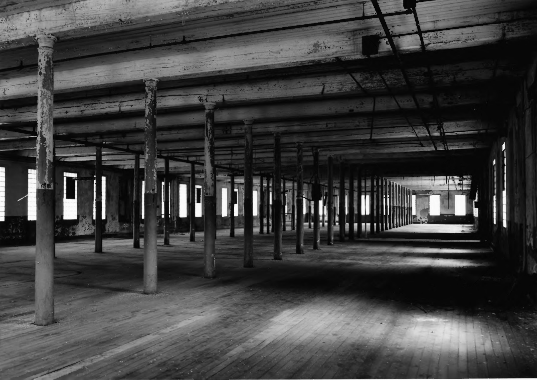
12. CANNELTON MILLS, INDIANA Third Floor, Westerly Direction Photo: Boucher, HAER, 1974
