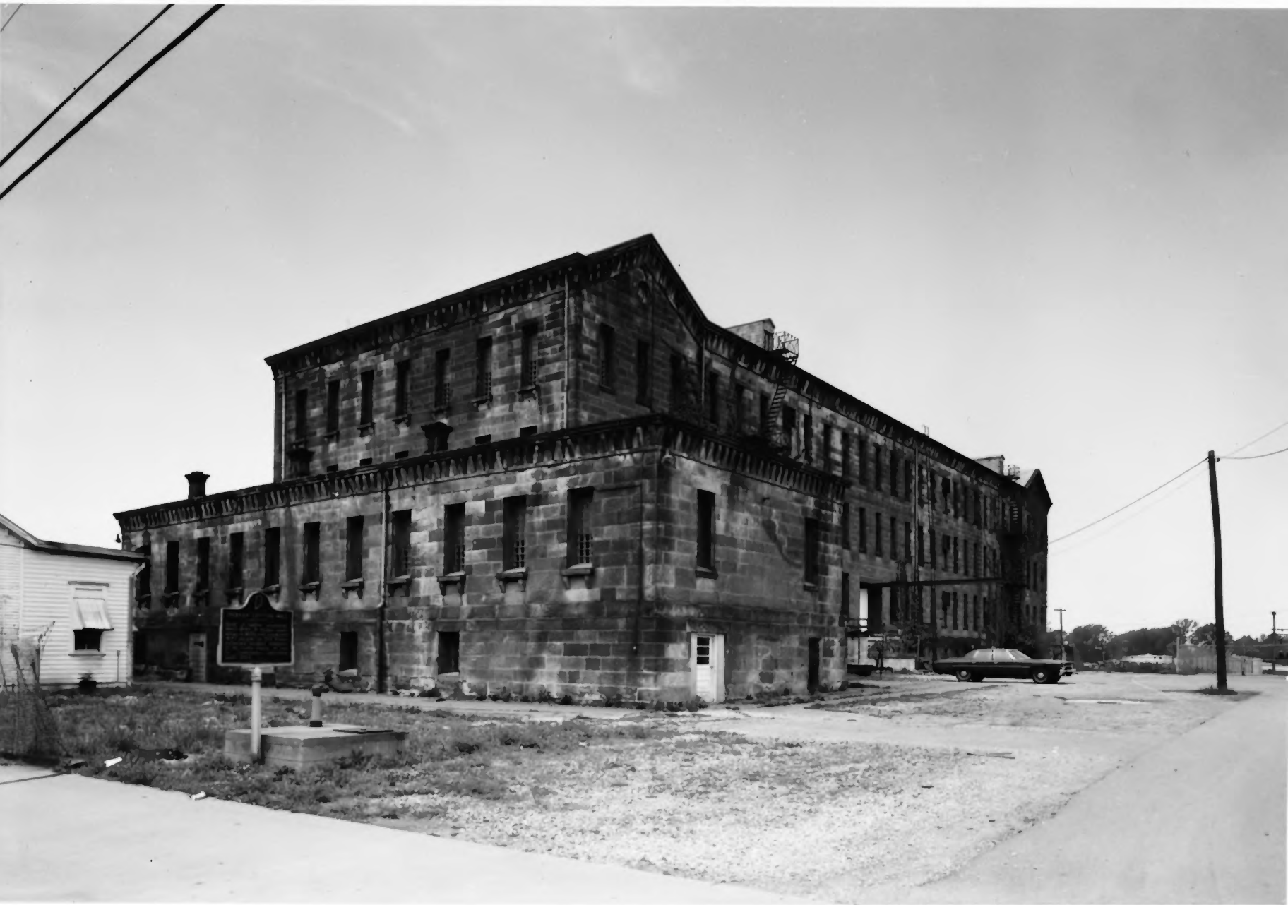
CANNELTON MILLS, INDIANA View of Southeast End Photo: Boucher, HAER, 1974
