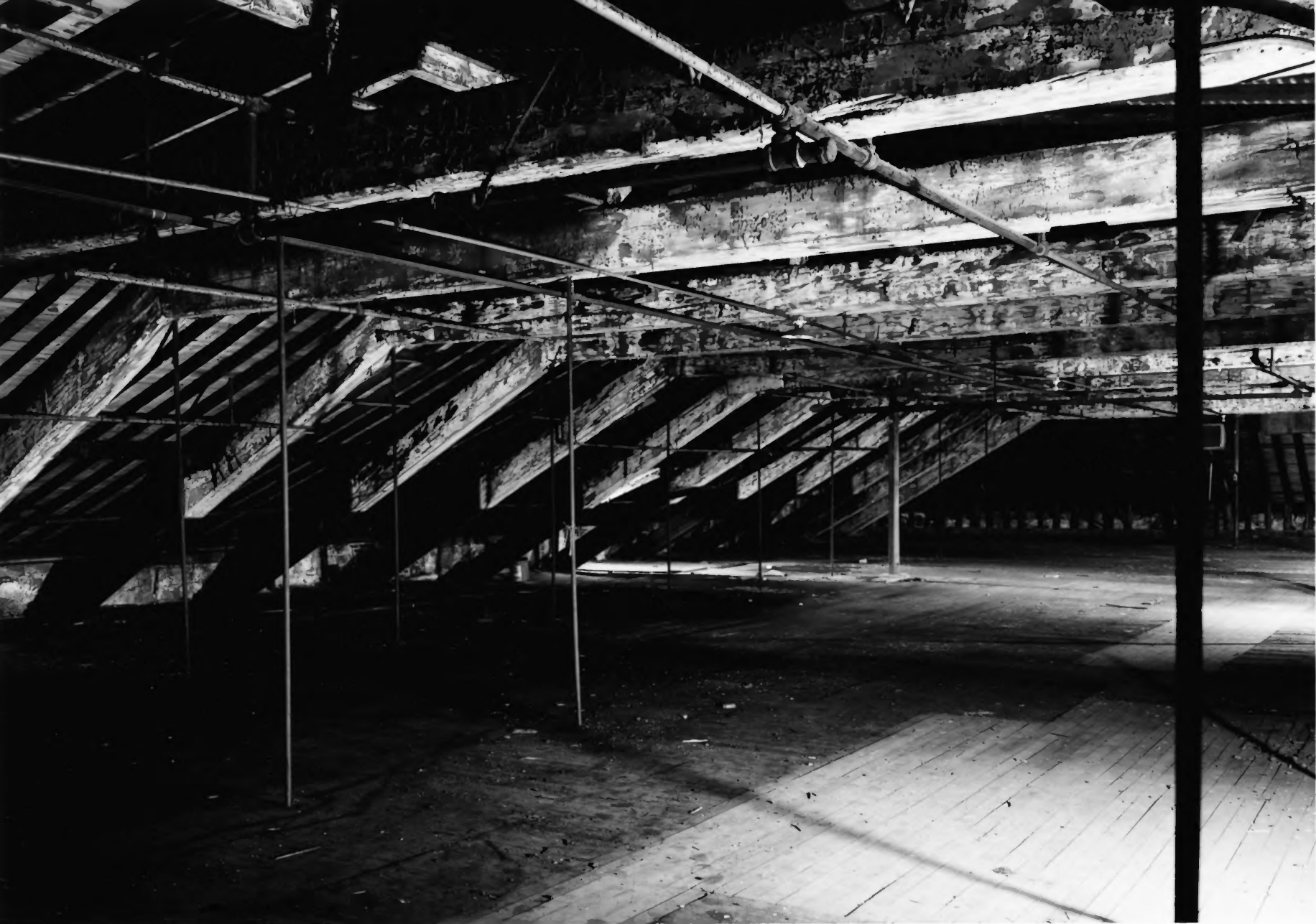
11. CANNELTON MILLS, INDIANA Attic Photo: Boucher, HAER, 1974
