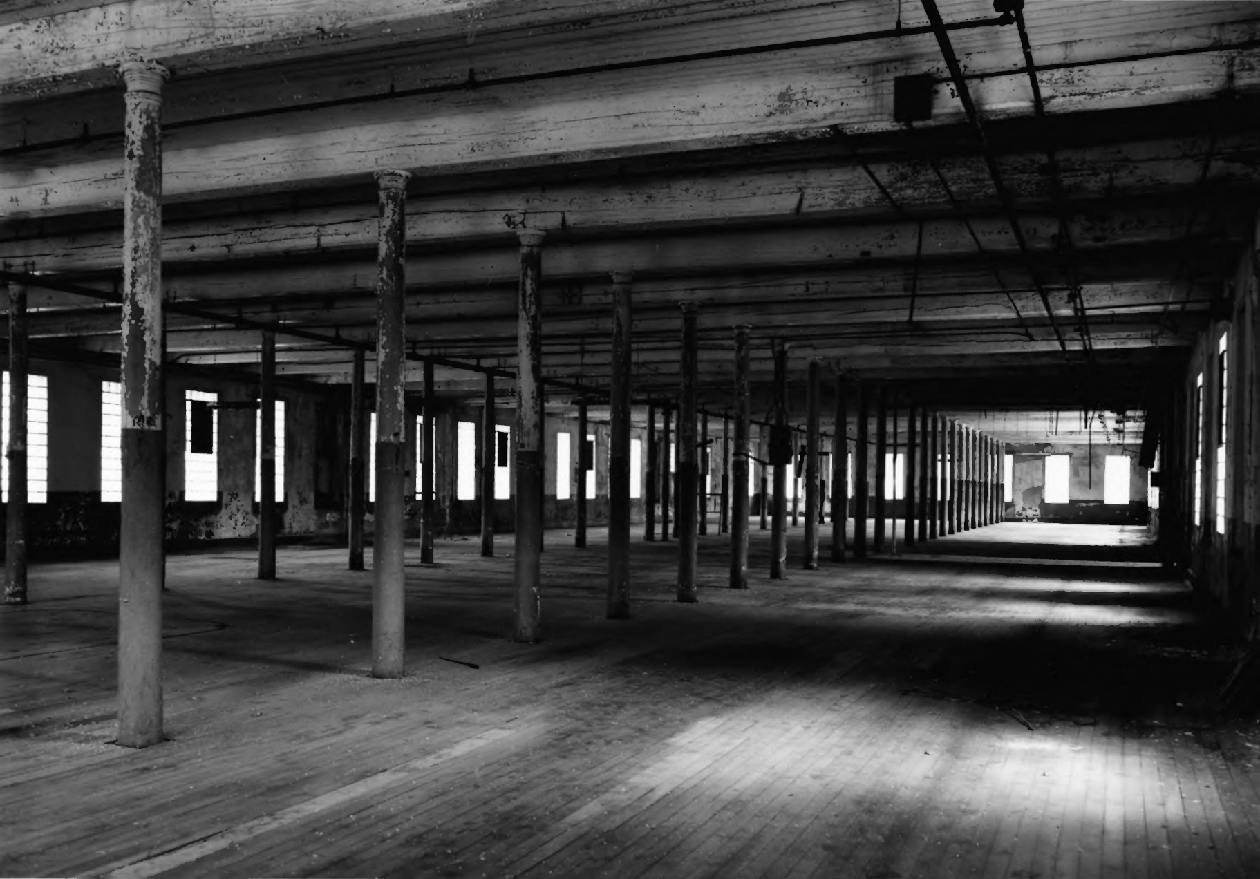
10. CANNELTON MILLS, INDIANA Third Floor, West Photo: Boucher, HAER, 1974
