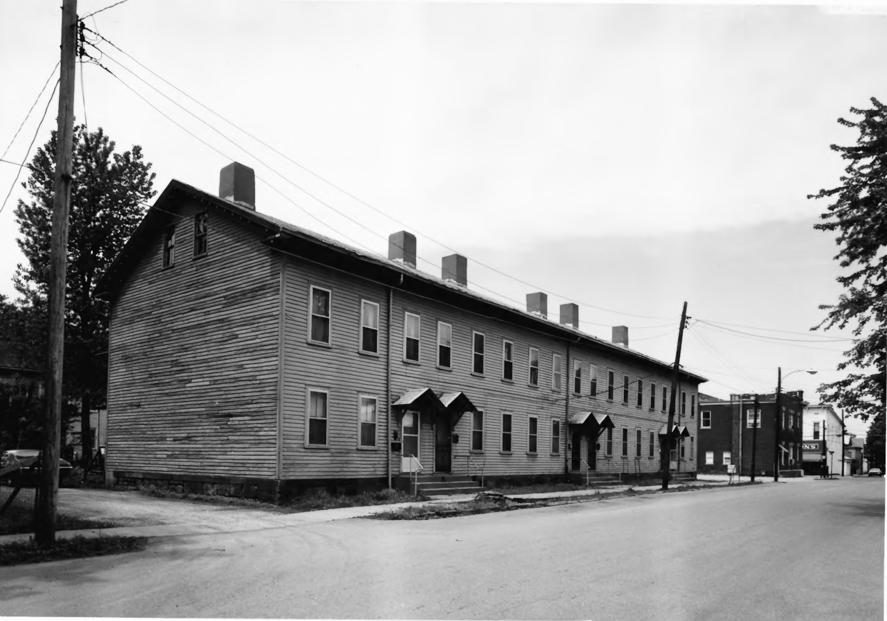
18. CANNELTON MILLS, INDIANA Workers' Housing Fifth Street Row From East Photo: Boucher, HAER, 1974
