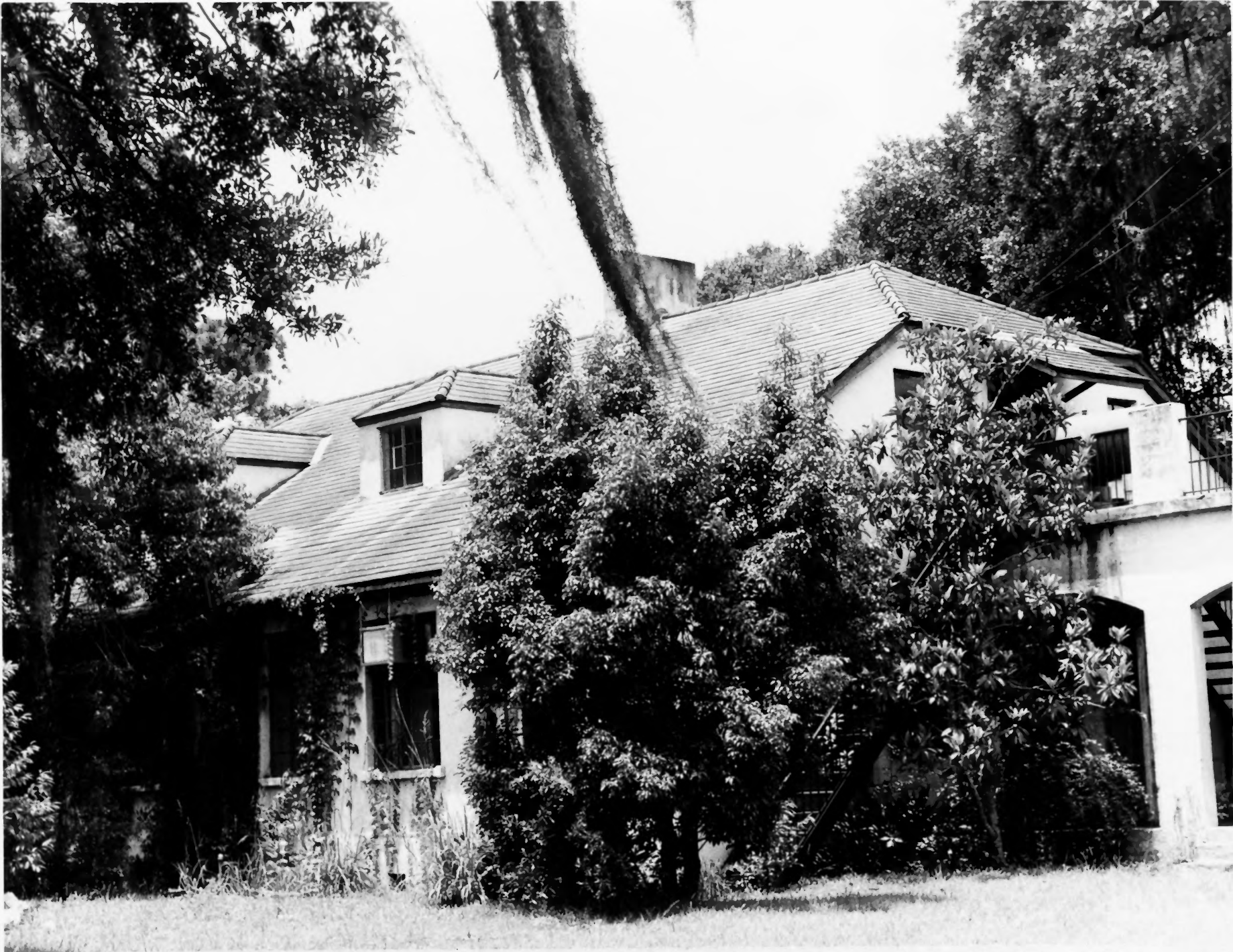
Butler Building, Penn Community Services, Fragmore, South Carolina
