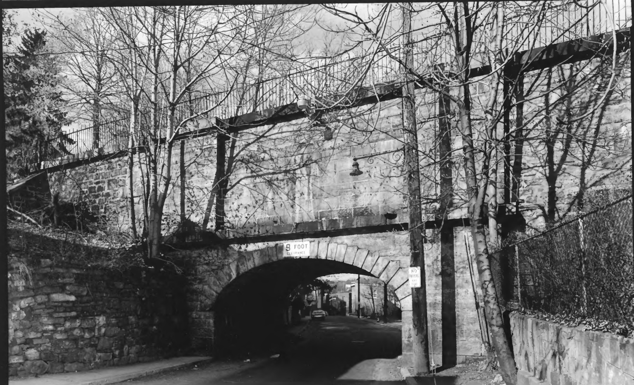
PHOTOGRAPH #15 Croton Aqueduct
