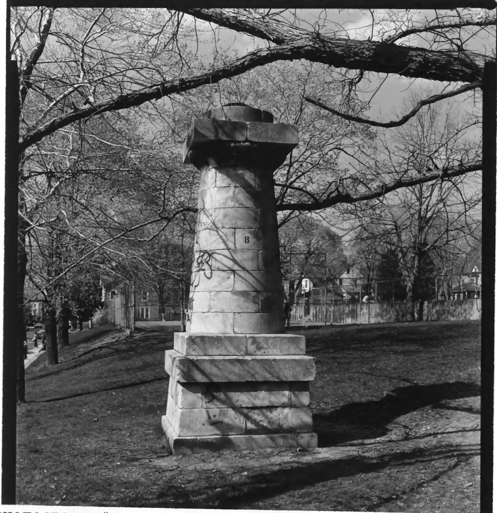
PHOTOGRAPH #5 Croton Aqueduct Ossining, New York Ventilator Shaft No. 9 at Spring Street and Everett Avenue. Jack Boucher, 1978, HAER Photo No. NY-111-1.
