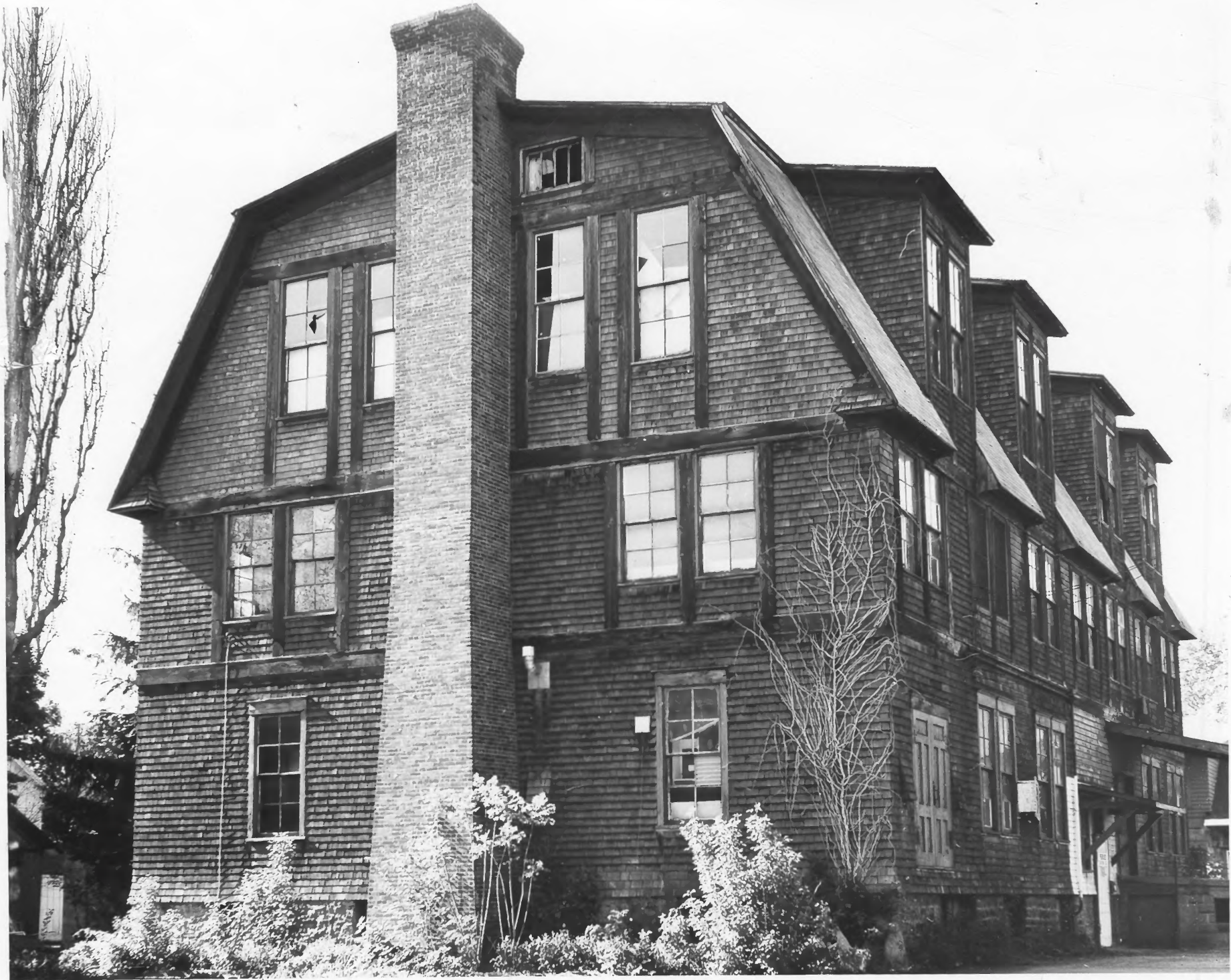
Roycroft Campus, view of Furniture Shop and Book Bindery, looking northeast, 1973 National Register of Historic Places photograph
