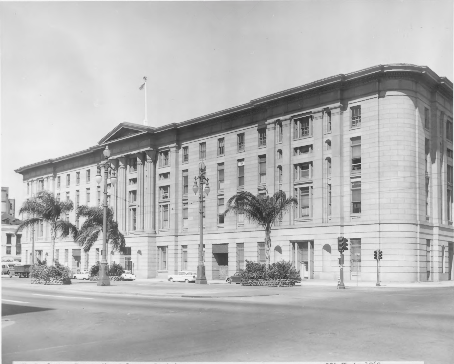
U. S. Custom House, New Orleans, Louisiana
