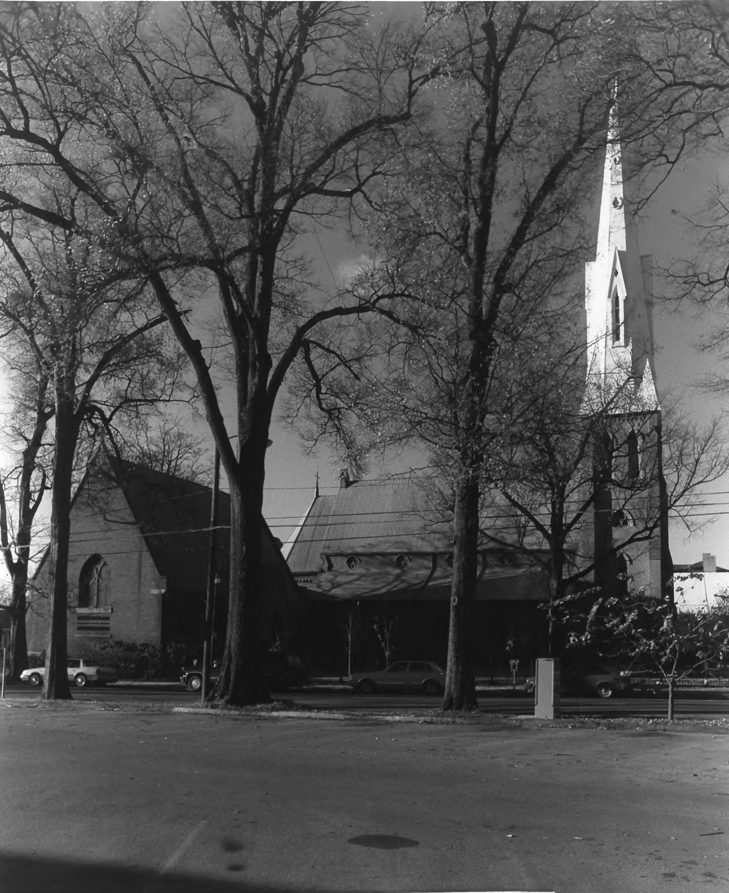
Church of the Nativity, Huntsville, Ala Photo: Harvie P. Jones, December, 1989 General view looking S, Bibb Chapel at left
