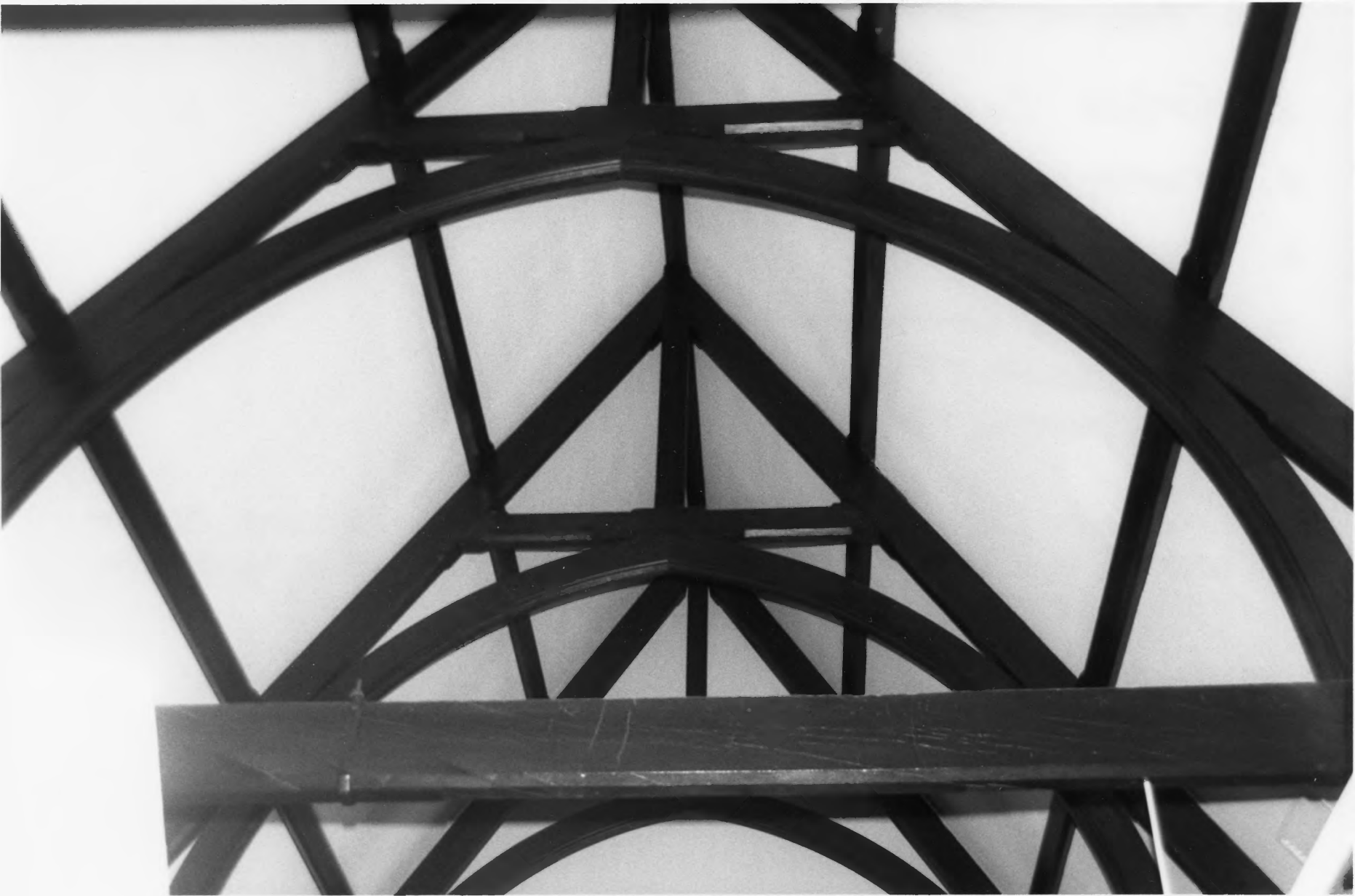
Adams Academy, Quincy, Massachusetts Interior ceiling, library Photo credit: M. Lehner 1993
