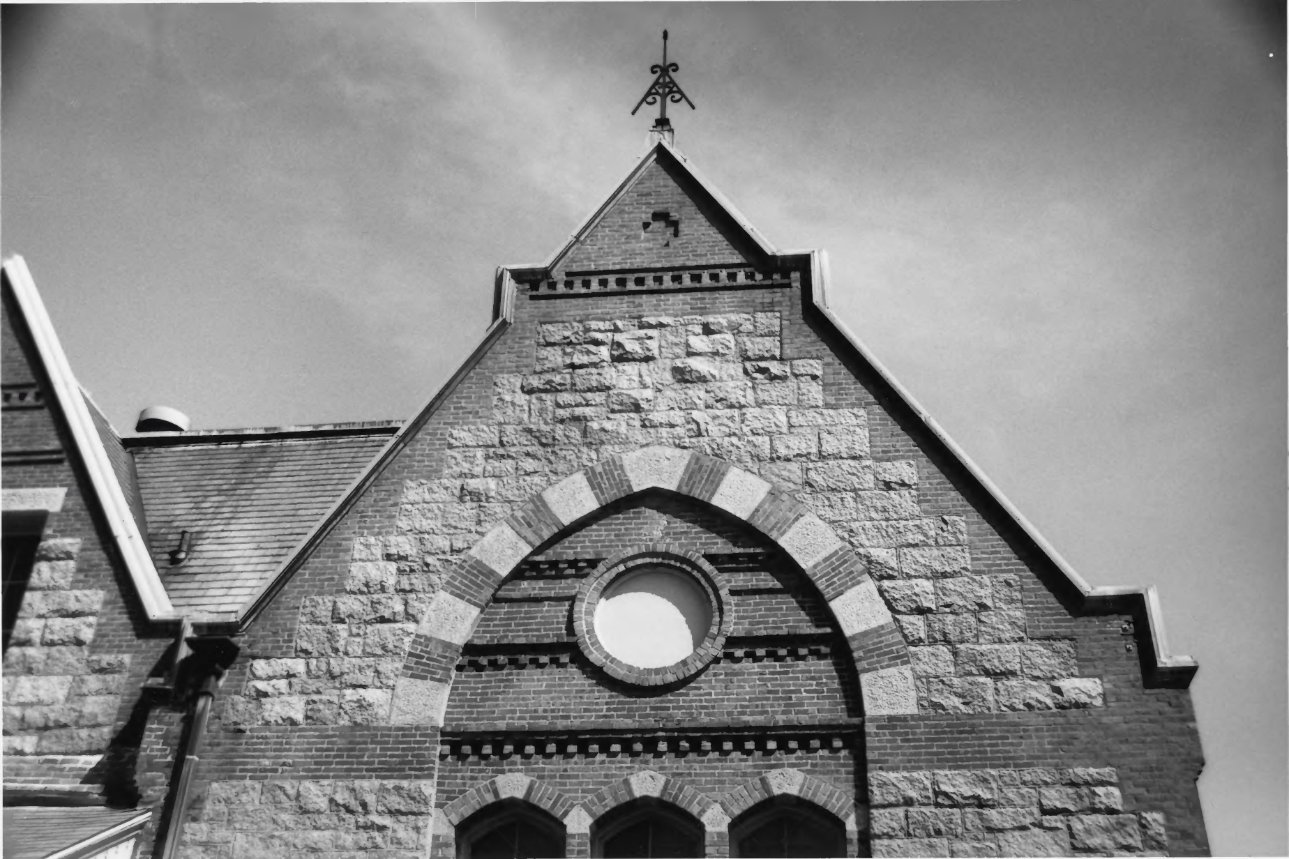
Adams Academy, Quincy, Massachusetts West elevation, gable Photo credit: M. Lehner 1993
