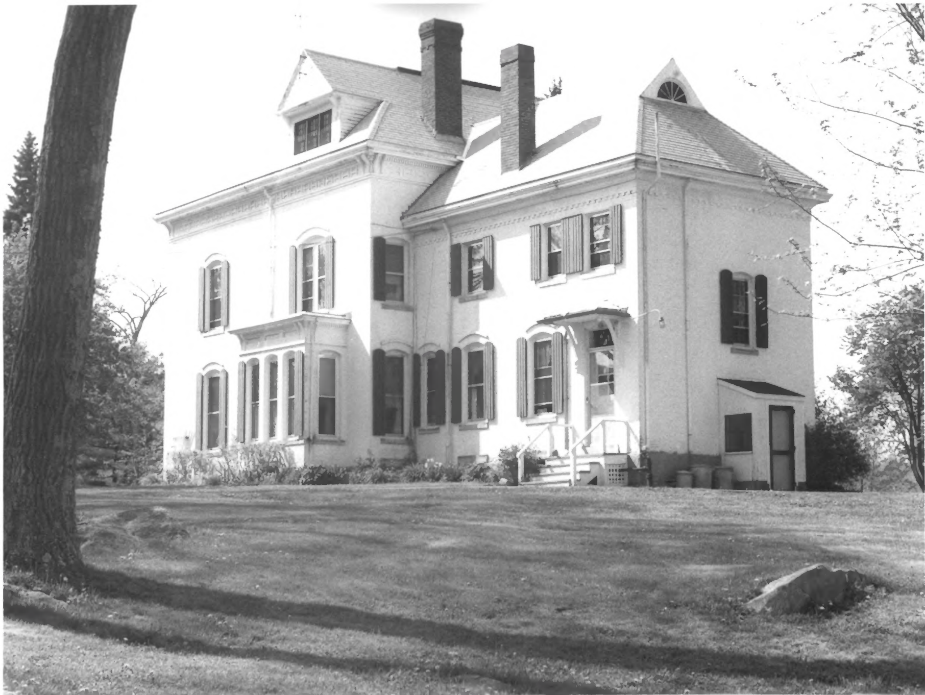
Treasurer's House (Building No. 3), National Home for Disabled Volunteer Soldiers, Togus Maine.
