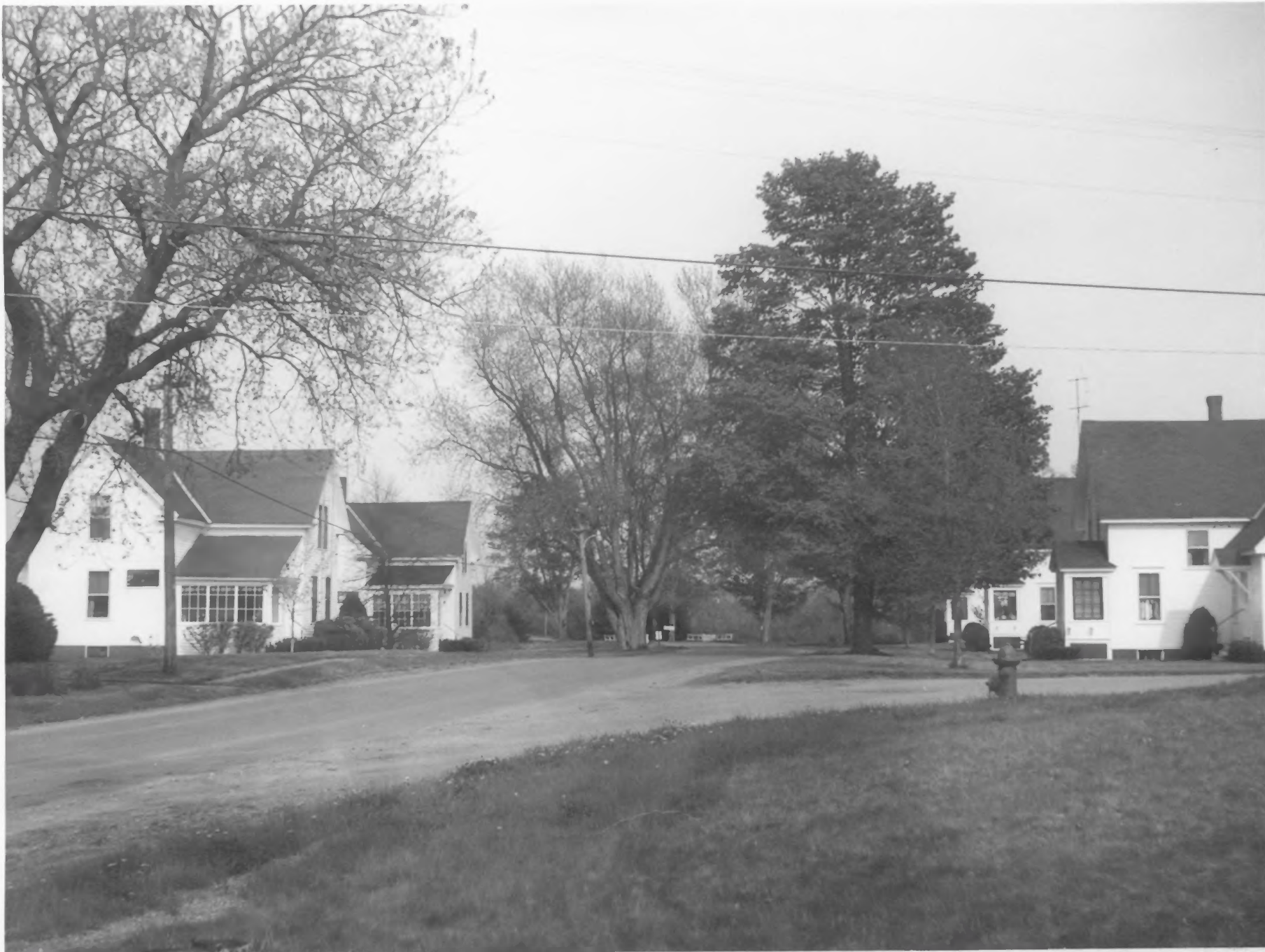
Employee Residence Cottages (Buildings 16, 17, 18, 19, 20), National Home for Disabled Volunteer Soldiers, Togus, Maine. NPS Photo 1973
