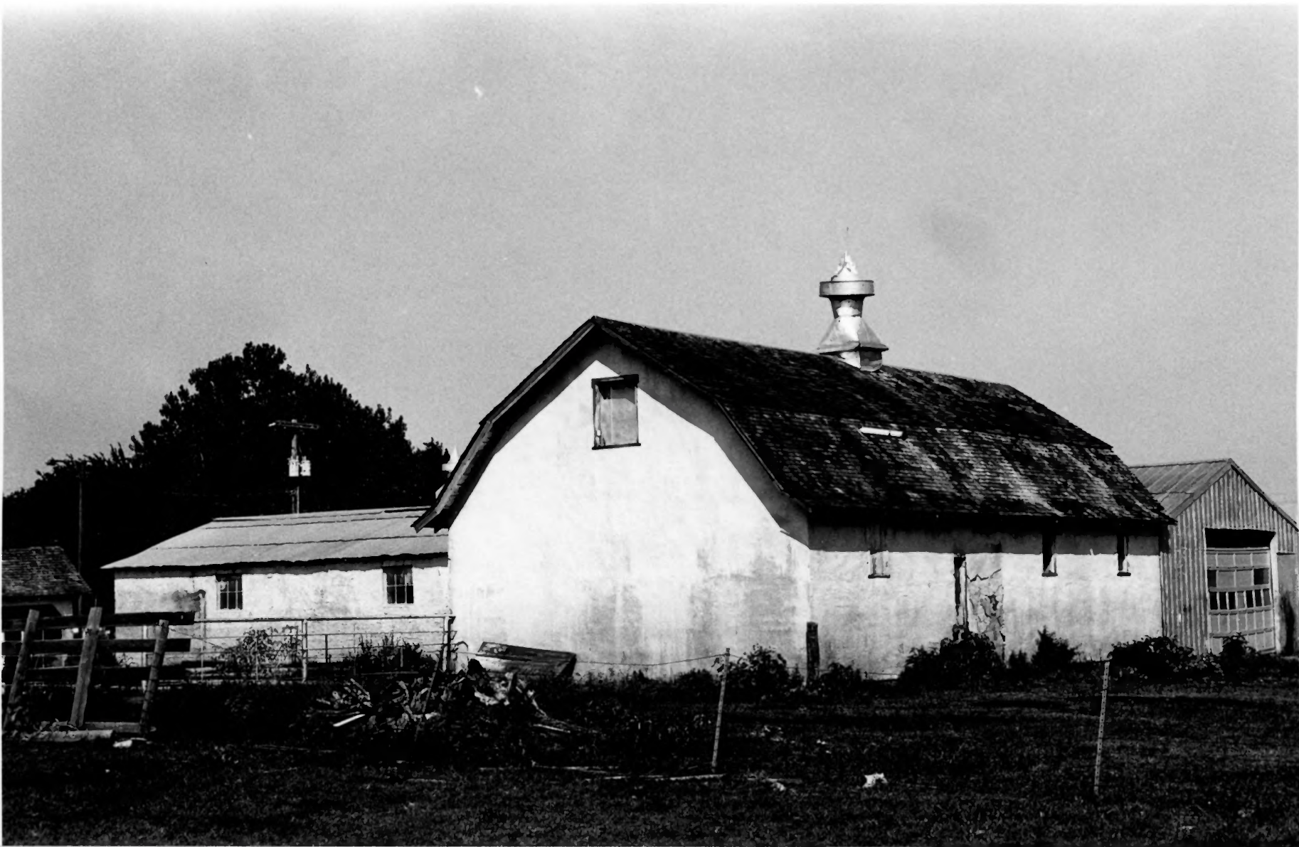
101 Ranch Historic District (Horse Barn), Marland, Oklahoma Photo by Peavler and Associates for ABC and NPS, 1974
