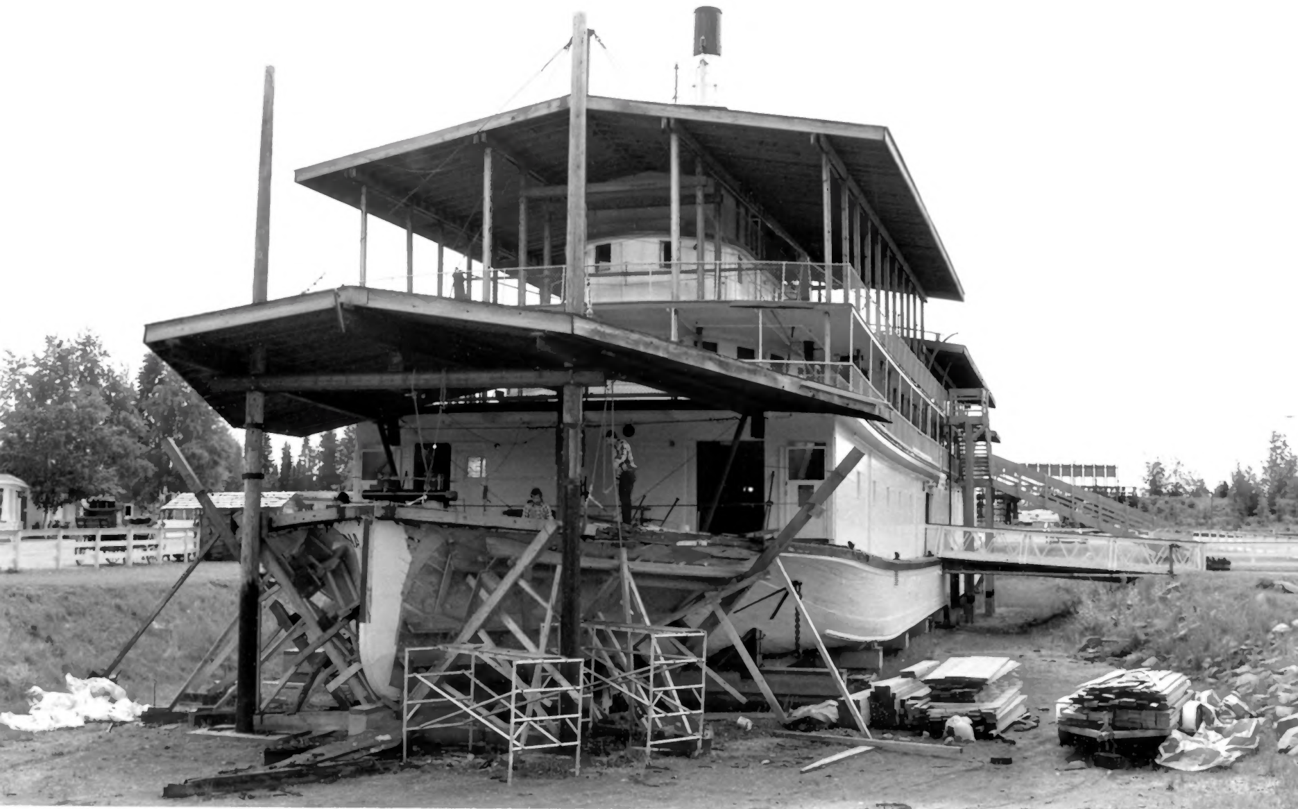
NENANA, Fairbanks, Alaska National Park Service Photograph by William S. Hanable, 1988 City of Fairbanks Port bow quarter view showing restoration work in progress, June 28, 1988. Photo #4
