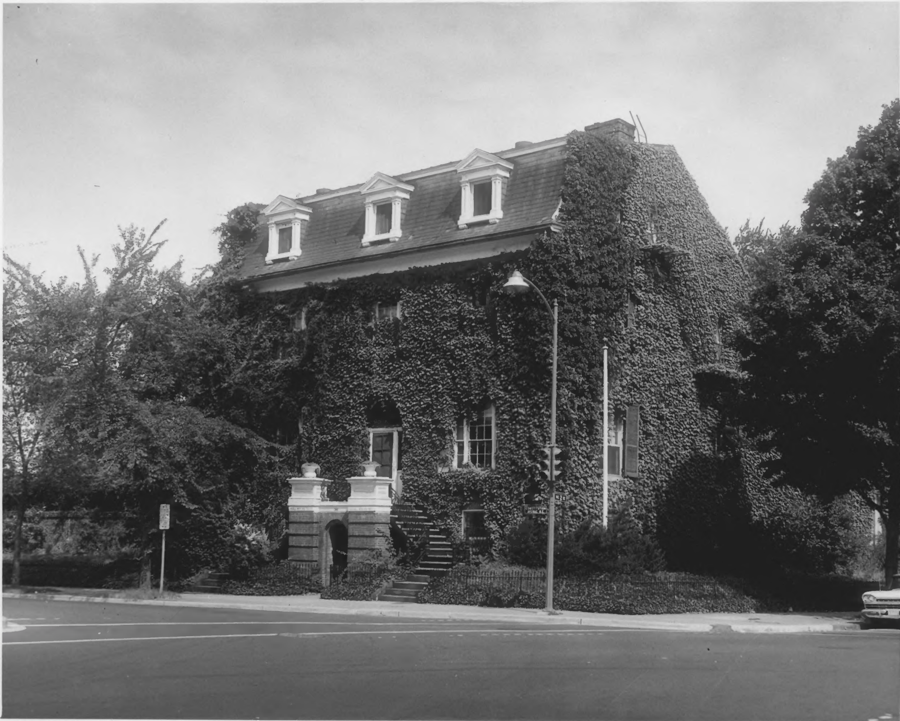
ALVA BELMONT HOUSE - 144 Constitution Avenue, N.E., Washington, D.C. South Front View. August 1961 - Photo-Courtesy of Abbie Rowe, National Park Service.
