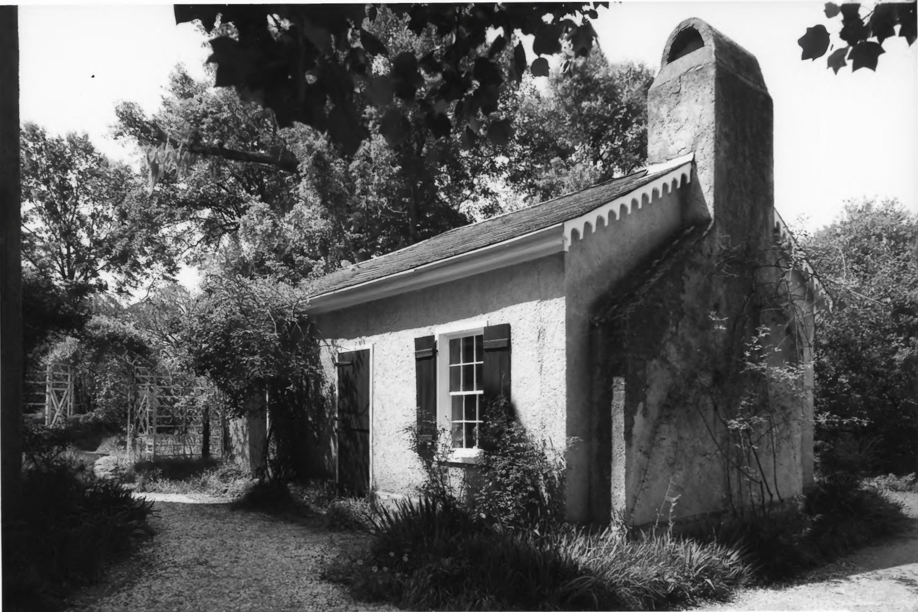
BOROUGH HOUSE: SUMMER KITCHEN - Stateburg, Sumter Co., South Carolina. GENERAL VIEW FROM NORTH. (HABS photo SC-366-5 by Jack E. Boucher, May 1985)
