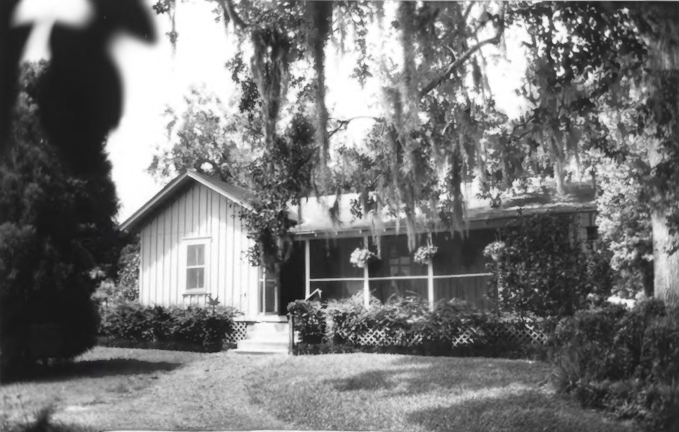
BOK TOWER GARDENS, Polk County, Florida. Photo 6: Rebecca Spain Schwarz, September 1992. Visitor Center: East elevation, looking southwest.
