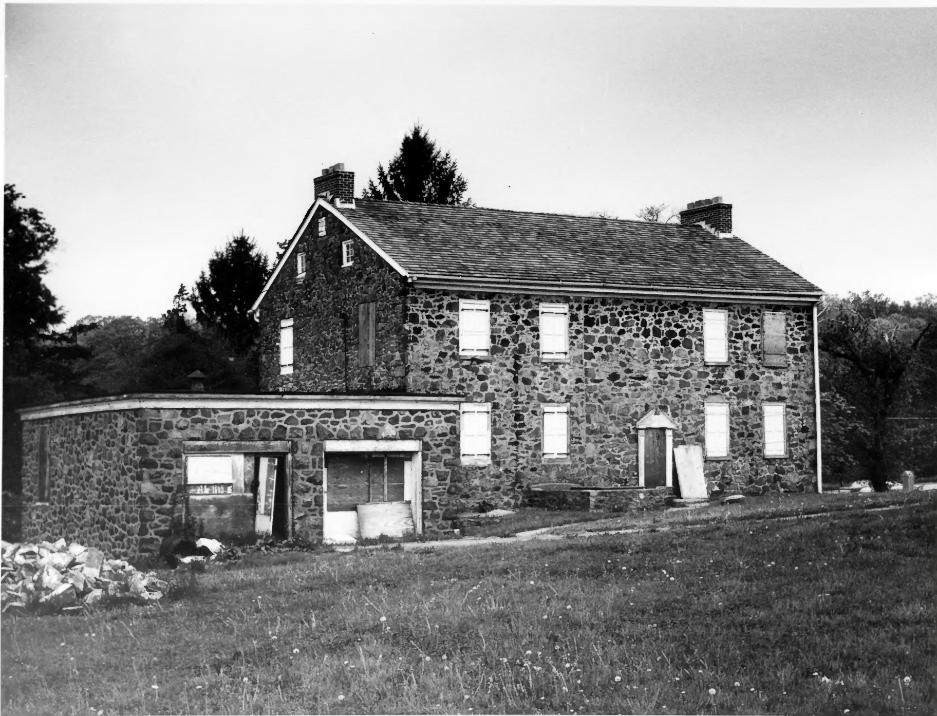
Gunning Bedford, Jr., House, (Lombardy Hall), Wilmington, Delaware
