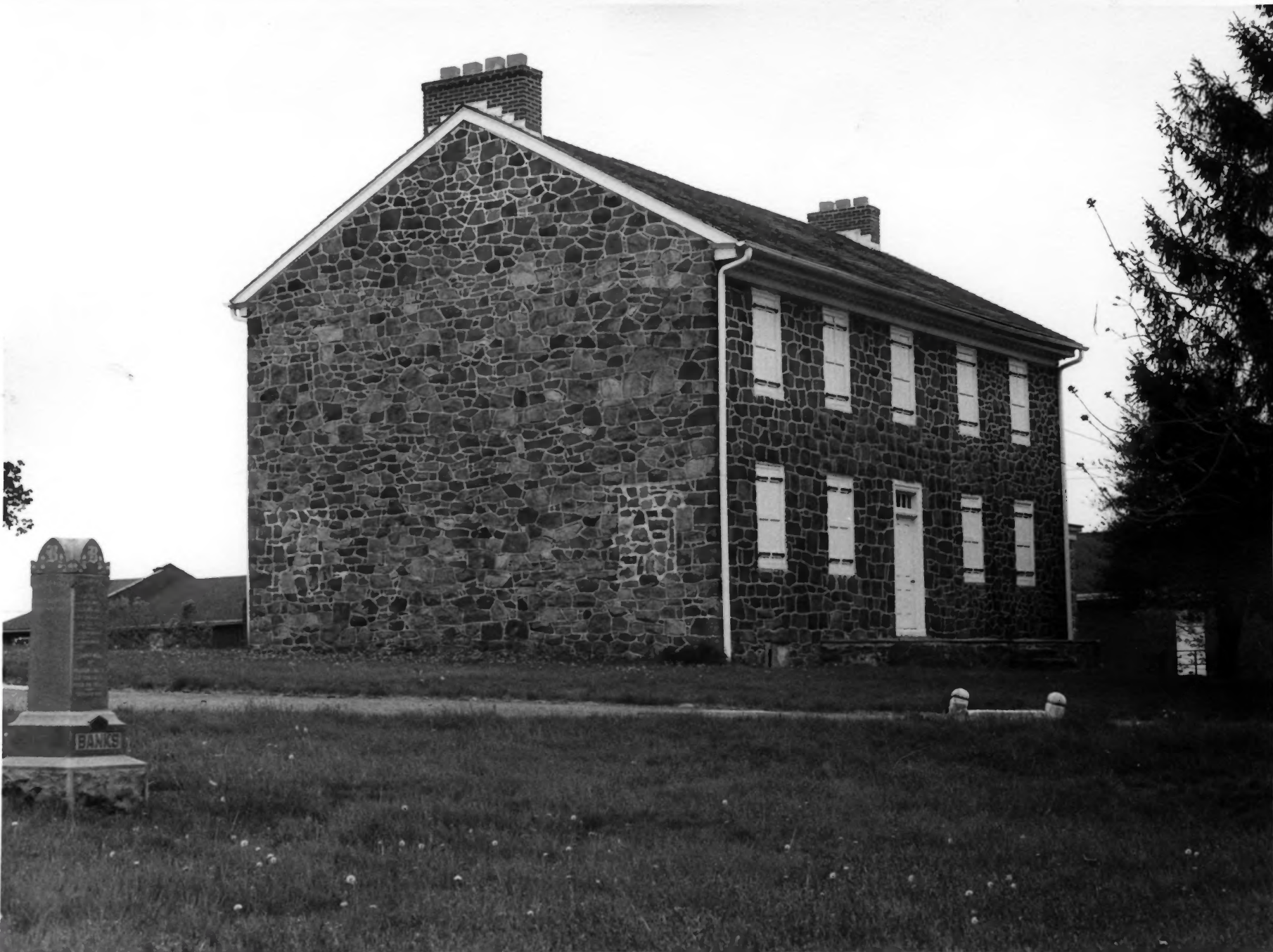
Gunning Bedford, Jr., House, (Lombardy Hall), Wilmington, Delaware
