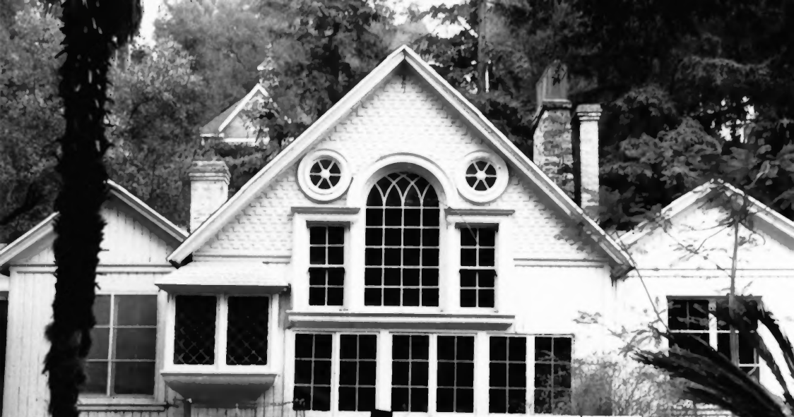
Modjeska House, Orange County California Main house, north facade, before stabilization Photo: Marshall Duell Orange County, 1988
