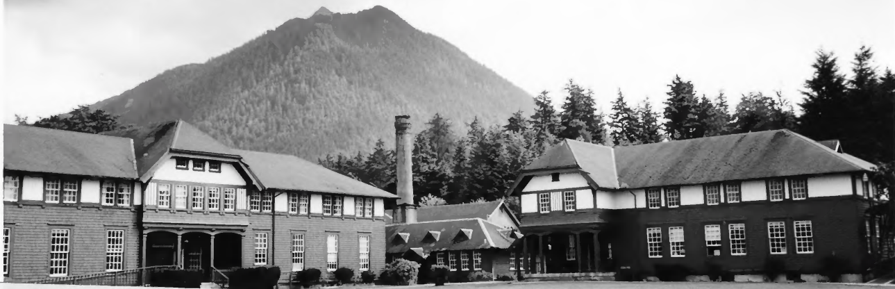
SHELDON JACKSON SCHOOL Whitmore Hall, Power Plant and Laundry, Fraser Hall (left to right) Sitka, Alaska Northeast view Photo by Amanda Zeman, 1998
