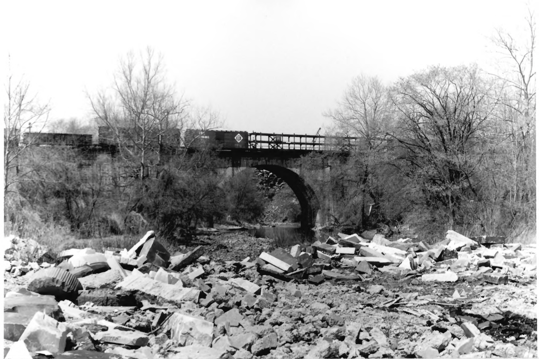
Carrollton Viaduct, Baltimore, Maryland
