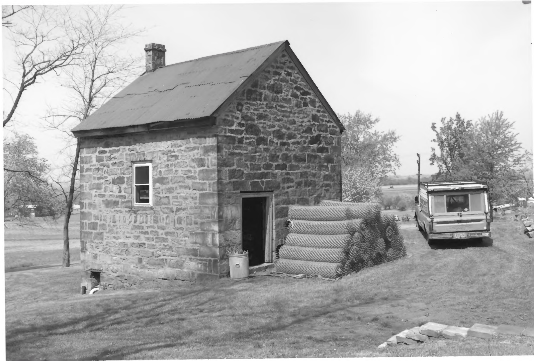
Isaac Meason House, Uniontown, Pa Photo: Jet Lowe. HAER 1989 5475/13 Smoke House, looking West
