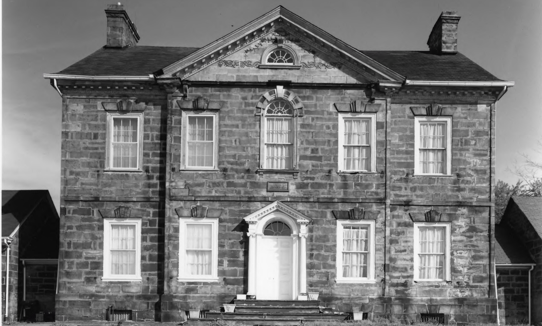
Isaac Meason House, Uniontown, Pa Photo: Jet Lowe. HAER 1989 5475/3 Main Block. Northwest front
