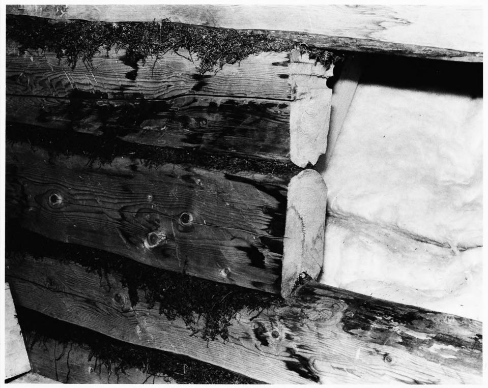
Holy Assumption Orthodox Church Kenai, Alaska Log detail, west end of nave wall (originally an outside wall) veiwed from second floor of bell tower through storage above entrance to name area
