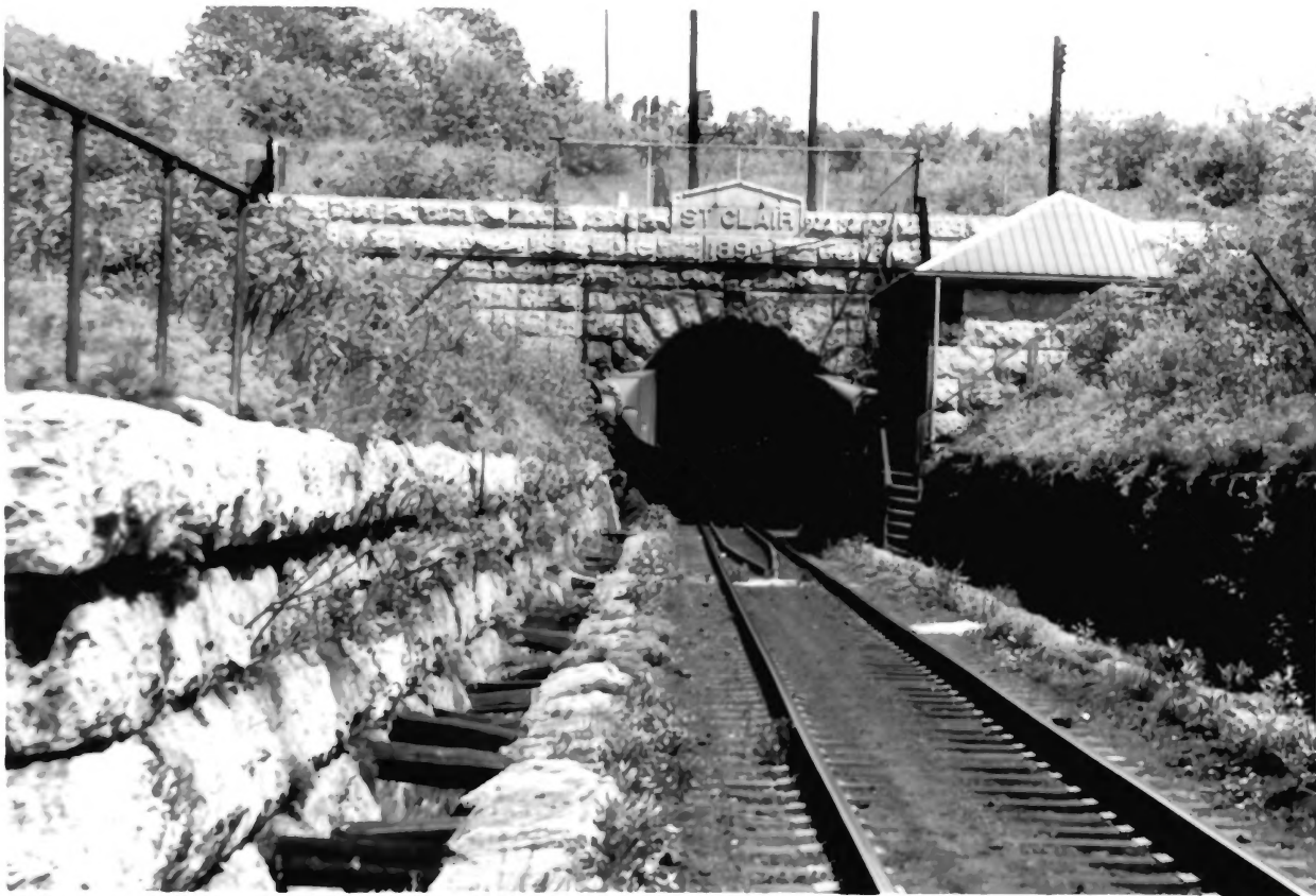
PHOTOGRAPH #1 St. Clair River Tunnel Port Huron, Michigan Port Huron Portal, Looking East Robie Lange, 1992
