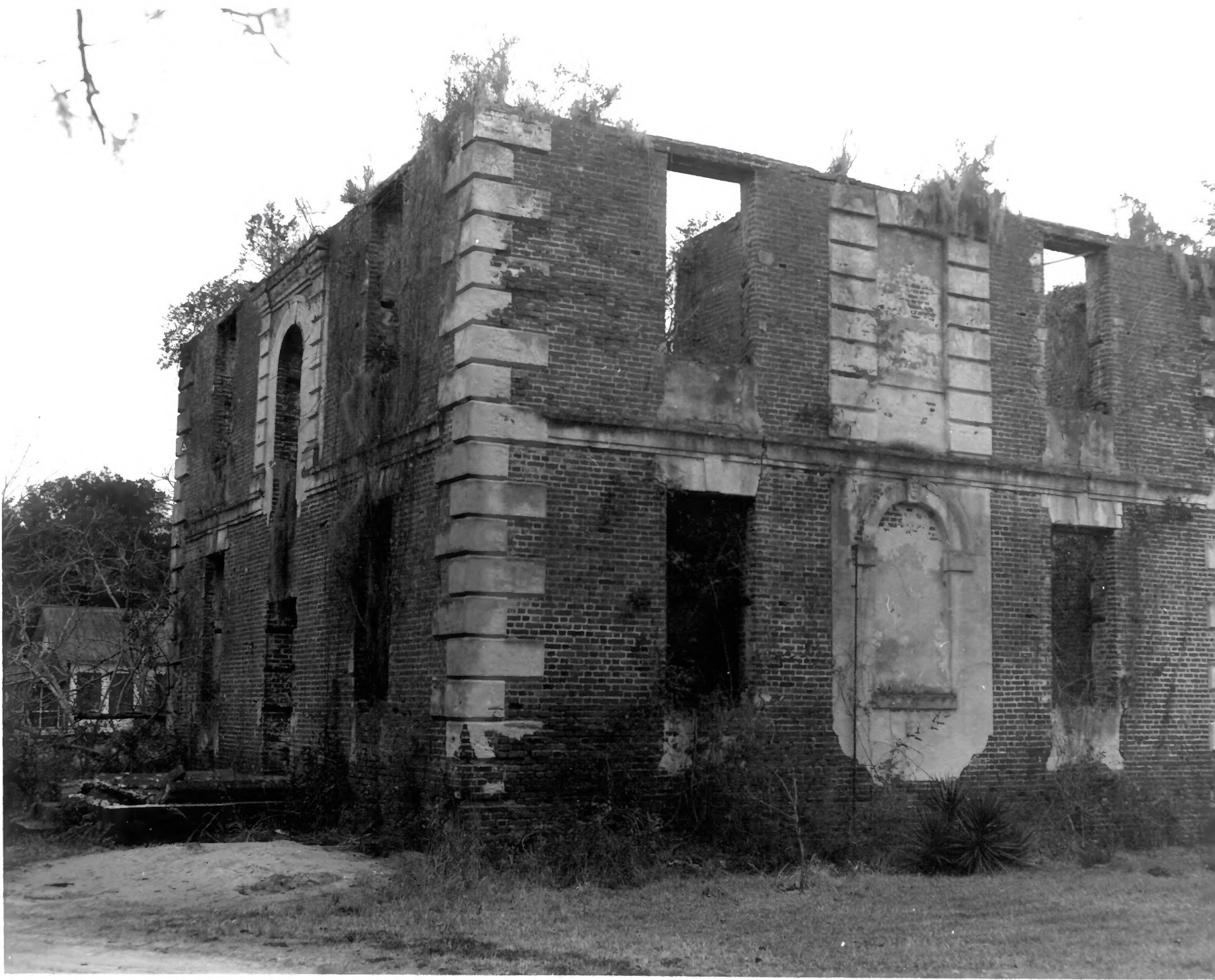
Brick House, west and north elevations, Edisto Island, South Carolina
