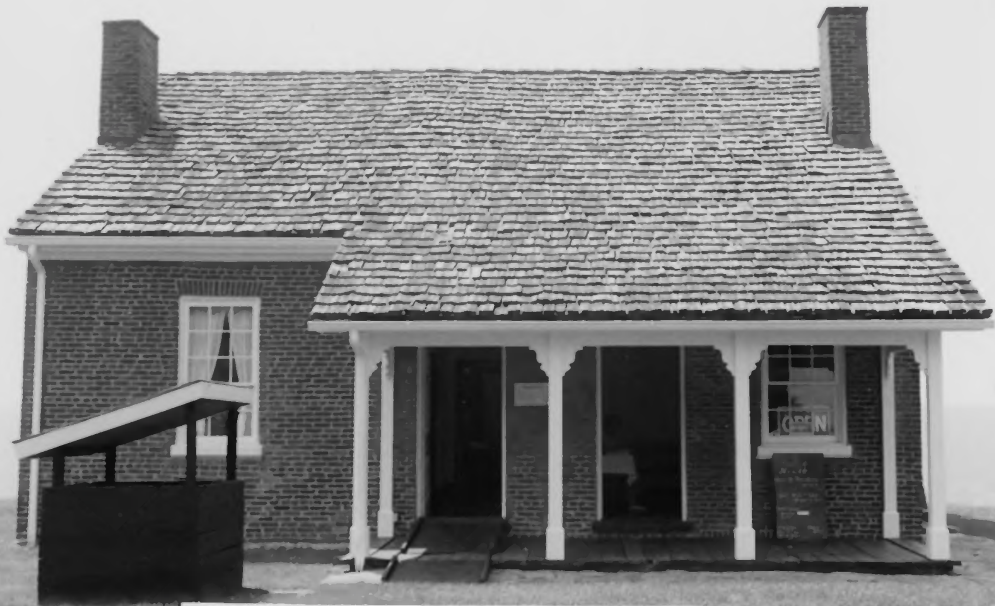
RANKIN, JOHN, HOUSE Ripley, Ohio North (rear) elevation Photo: Scott Roth, 1996
