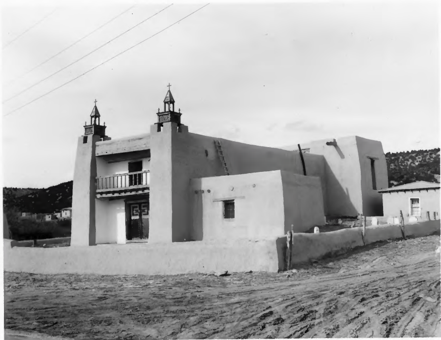
San Jose De Gracia Church, 1760-76 South (Front) Elevation, left; East Side, right on the north side of the Plaza at
