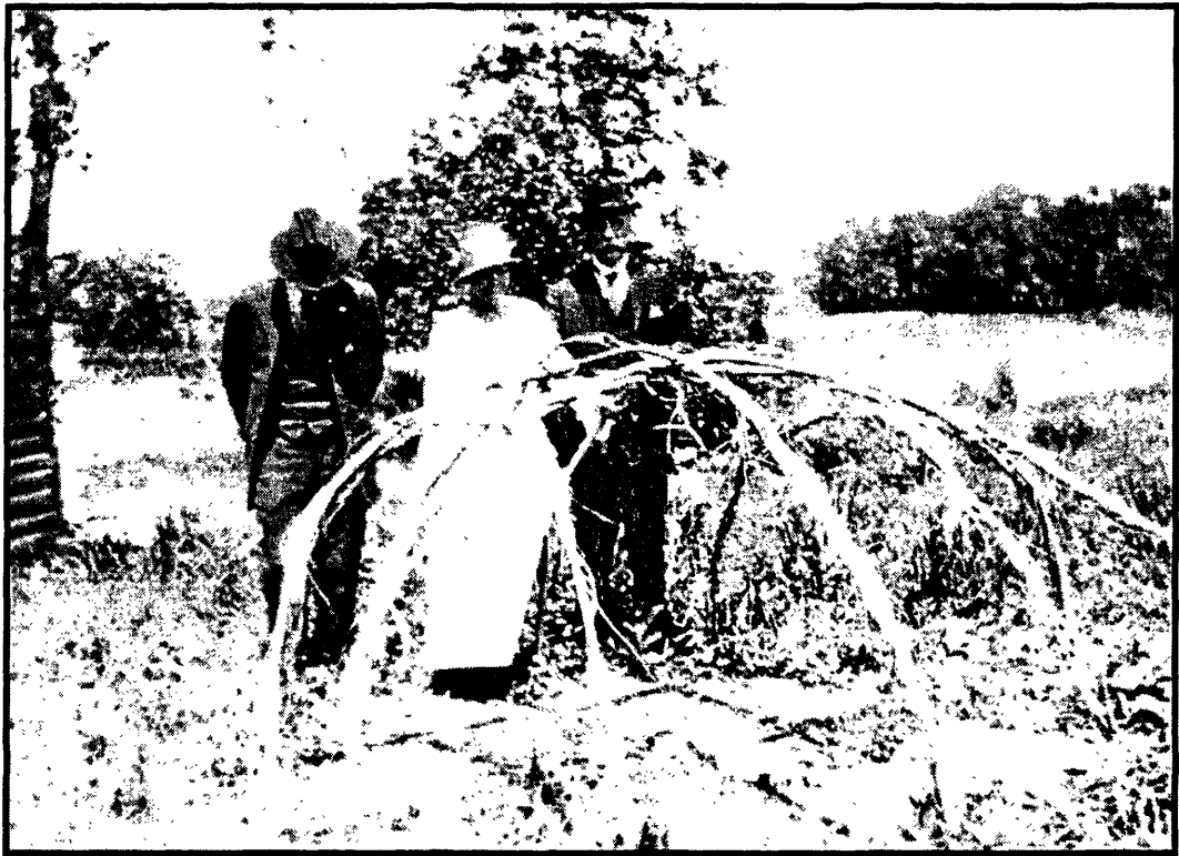
Figure 16. A frame for a sweat lodge near Plenty Coups' spring is being examined by visitors in this undated (circa 1920s) view. An edge of the small frame structure which covered the spring is shown at the extreme left. A caption on the back of the photograph reads: "A sweating bower for turkish baths, covered with mats, etc., steam from heated stones in the middle." SOURCE: Chief Plenty Coups Museum, Chief Plenty Coups State Park, Pryor, Montana, Photographic Collection, Image PAc82-26, Scrapbook II, p. 49, from an image in the Montana Historical Society, Helena, Montana.
