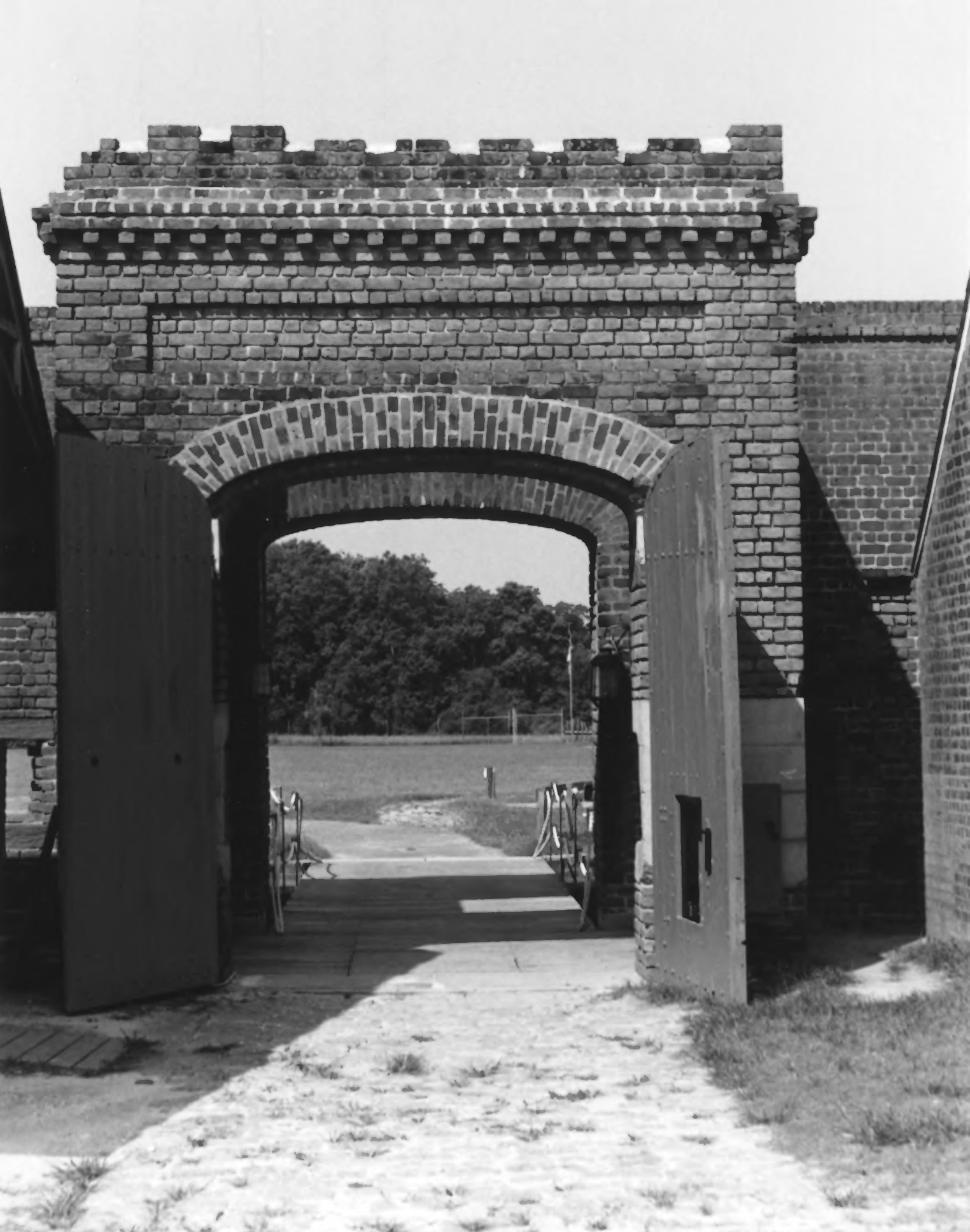
FORT JAMES JACKSON Chatham County, Georgia Sally port from interior, looking west Photo by Jefferson C. Reed, 1998
