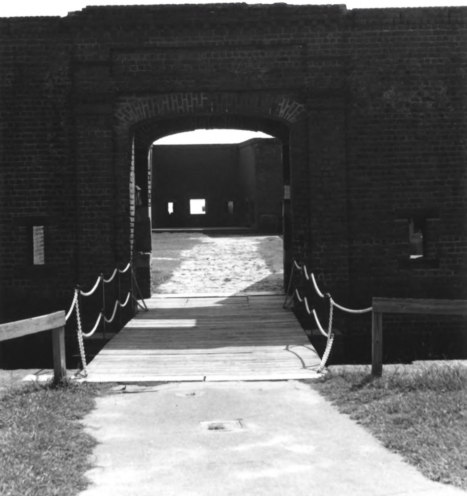
FORT JAMES JACKSON Chatham County, Georgia Sally port exterior, looking east Photo by Jefferson C. Reed, 1998
