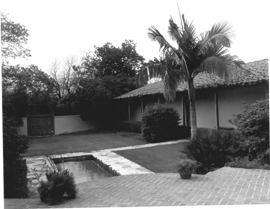
Los Cerritos Ranch House, 1844 West (Rear) Gate--Patio and North Service Wing (South Elevation)
