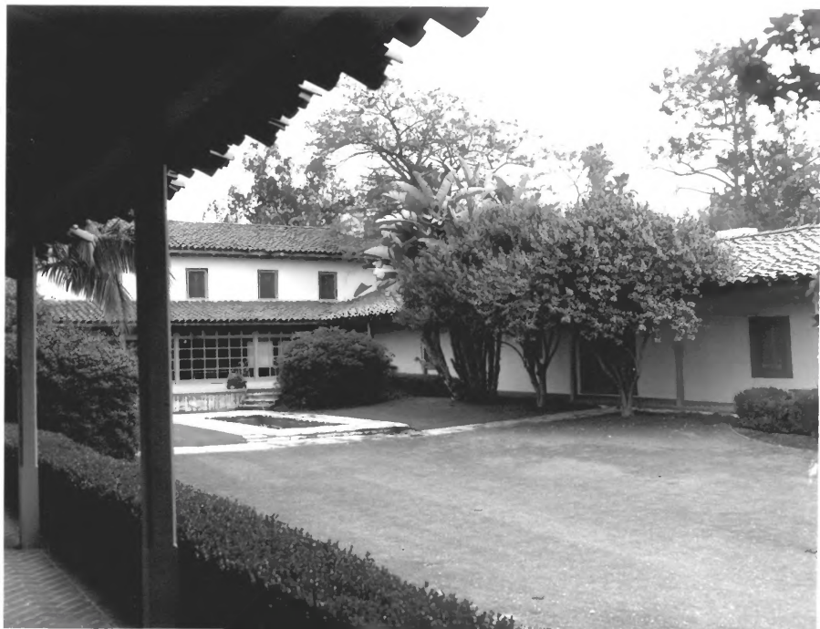
Los Cerritos Ranch House, 1844 West (Rear) Elevation of main house and north elevation of south service wing
