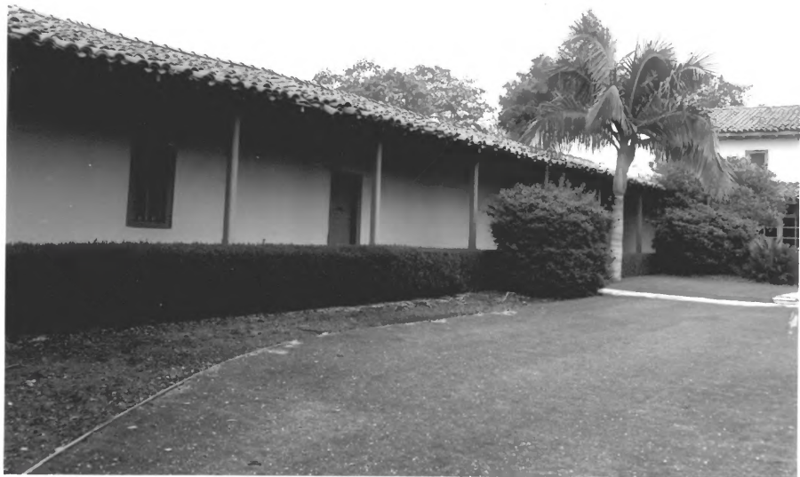
Los Cerritos Ranch House, 1844 South elevation of North Service Wing and West (Rear) elevation of Main House (Right)
