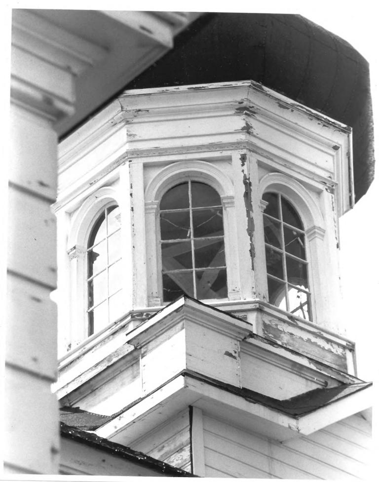
detail of tower, showing bracing beams and cupola
