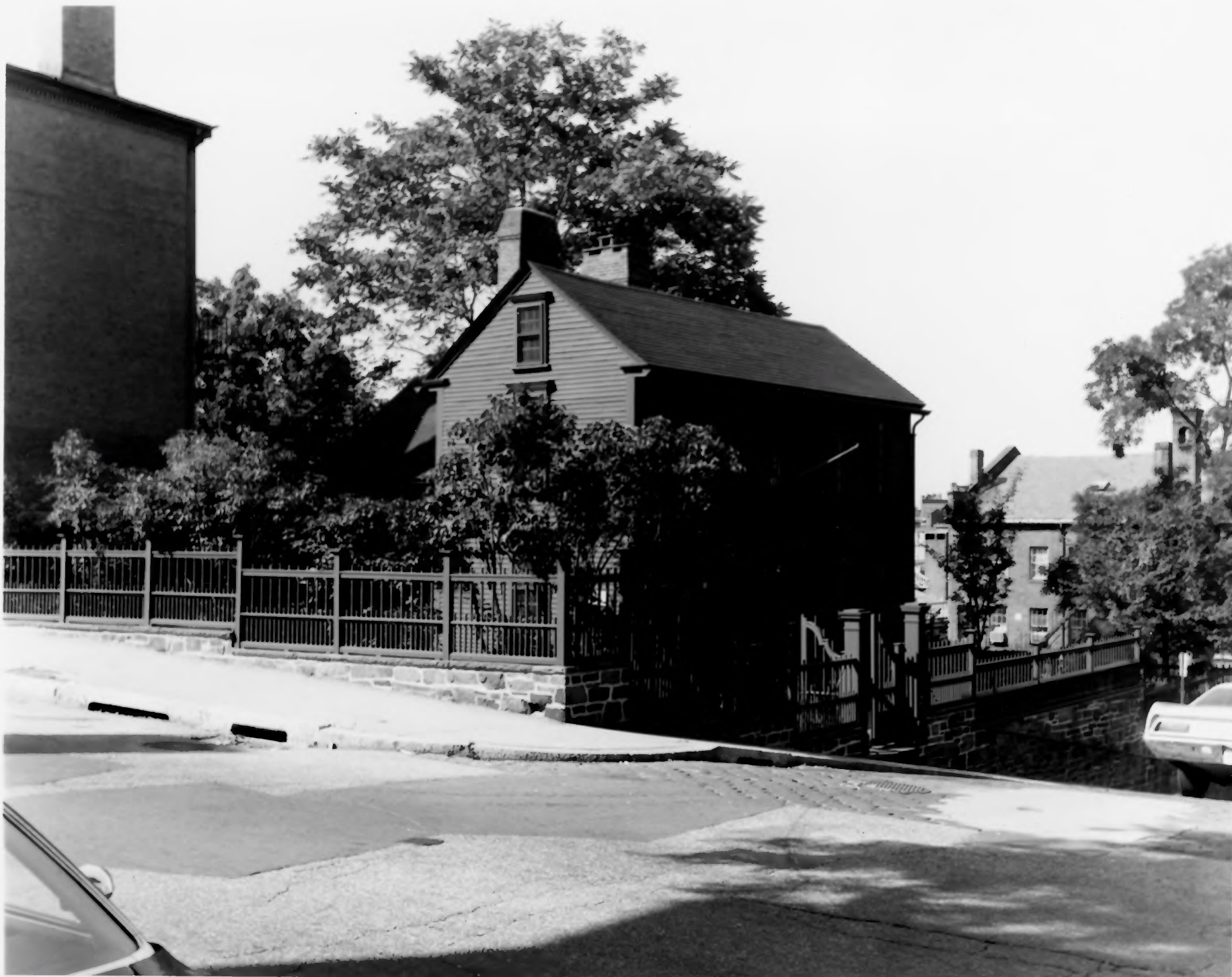
Gov. Stephen Hopkins House, Providence, Rhode Island
